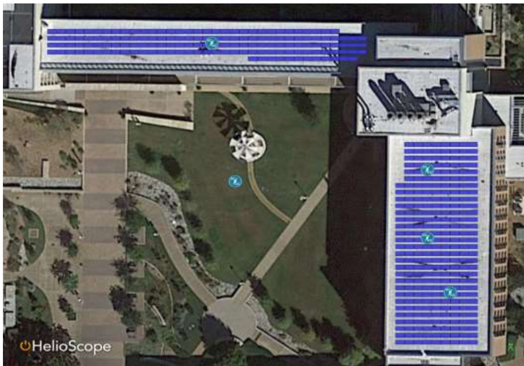
Figure 12. Aerial photo with designed solar panels at the Engineering Research Building (ERB)
