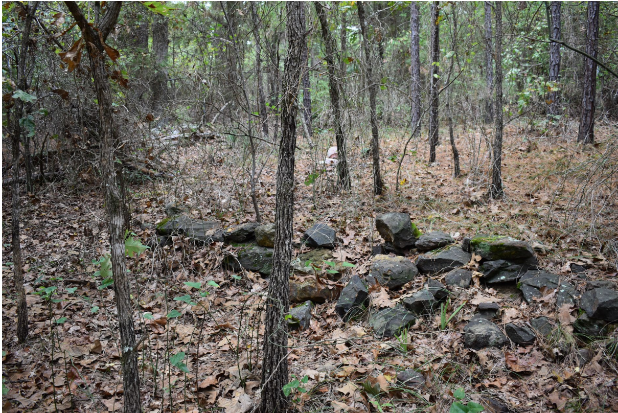
Figure 4-16 Retaining wall deteriorating
