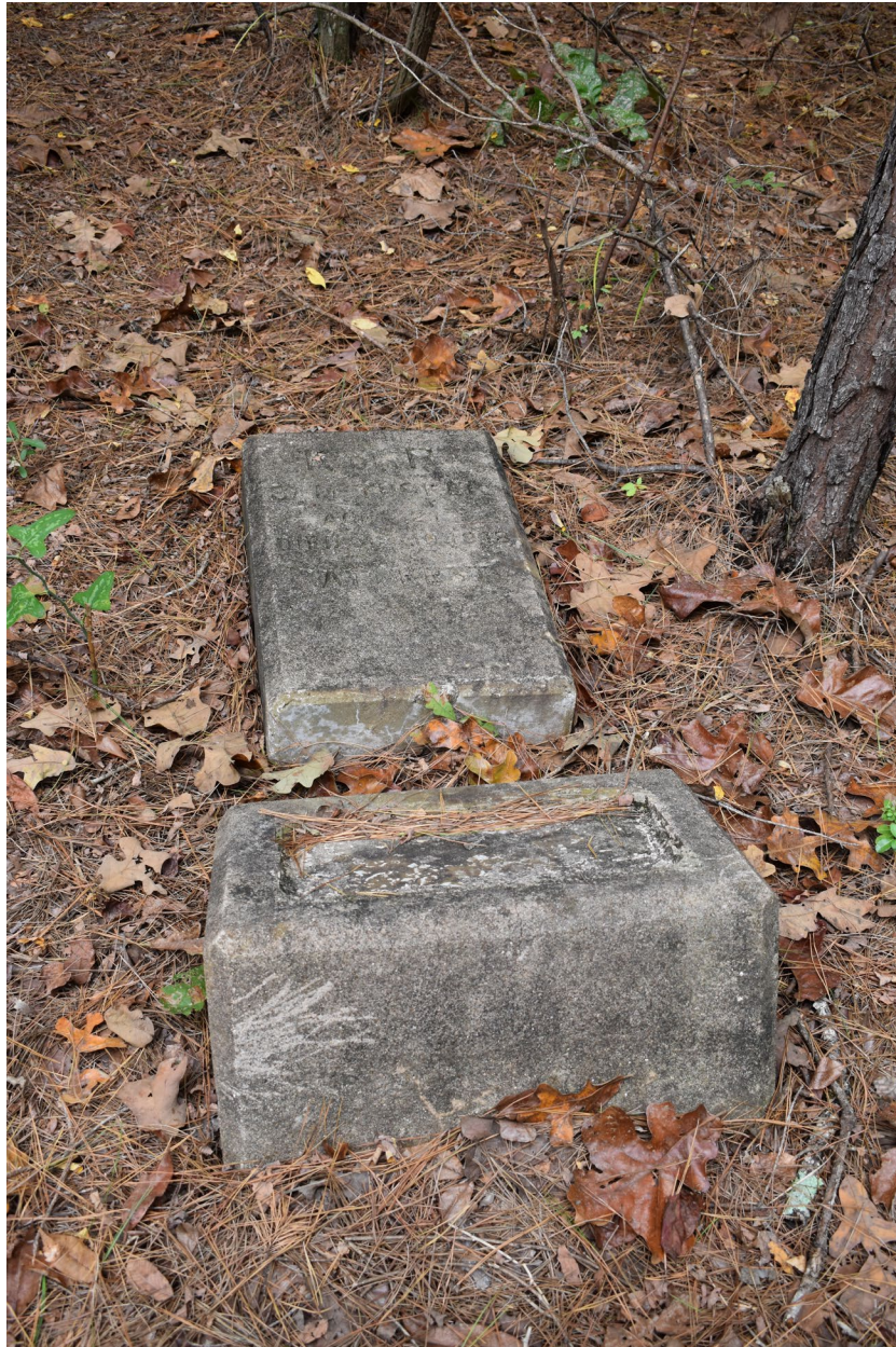
Figure A-12 Headstone needing to be repointed
