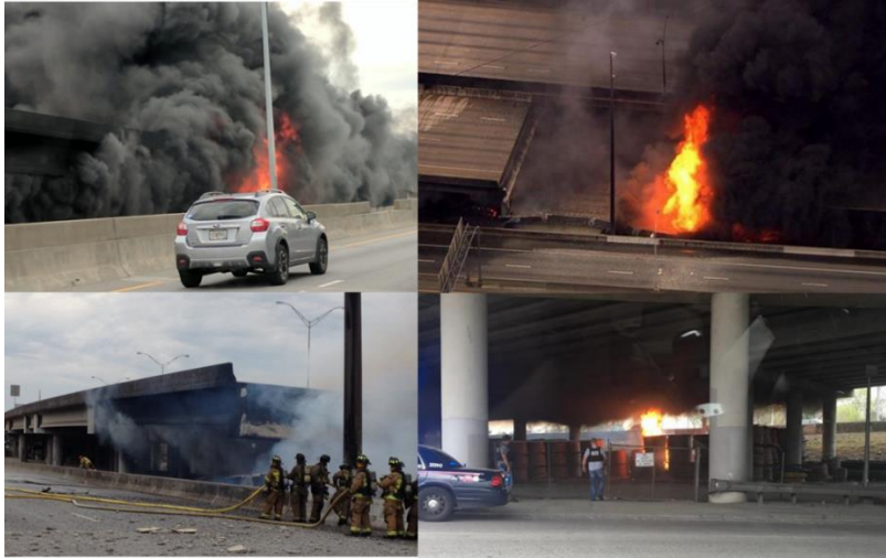
Figure 1- 5: Fire incident under a bridge on I-85 in Atlanta (Atlanta News, 2017).
