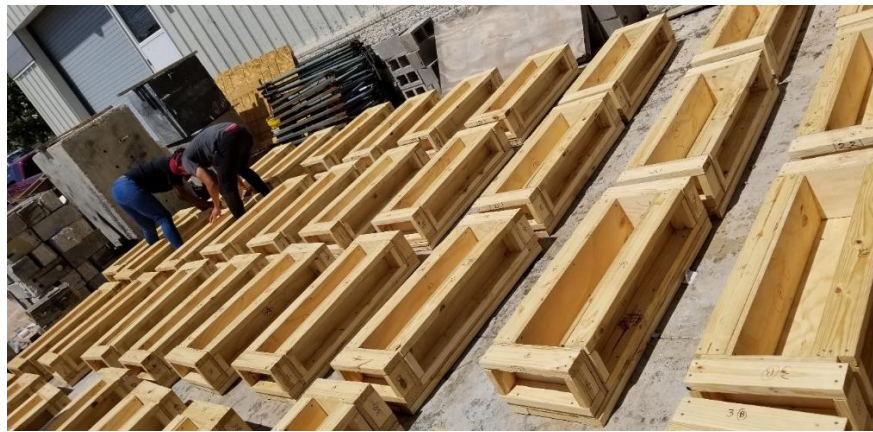
Figure 3- 4: Formwork preparation and laying for the main study.
