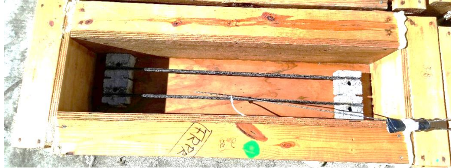
Figure 3- 5: Rebar placing in the formwork for the main study.
