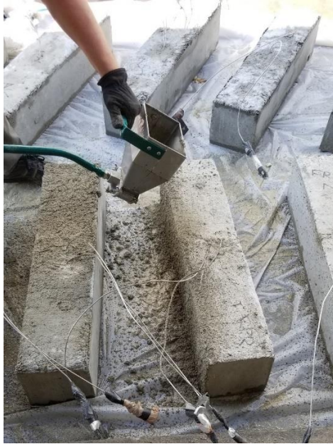
Figure 3- 8: Applying fireproofing mortar by spray or shotcrete.
