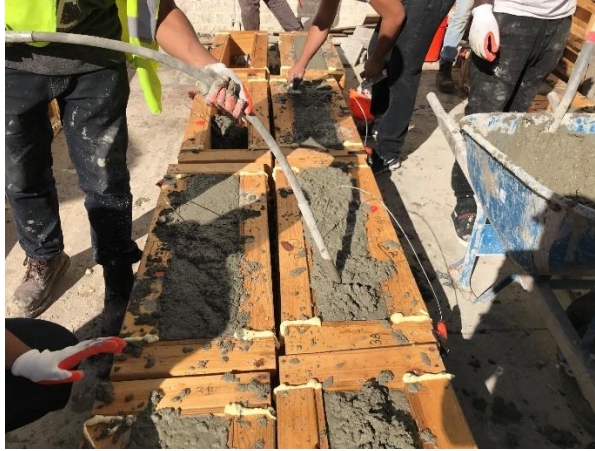
(a) Casting beam samples for the main study.
