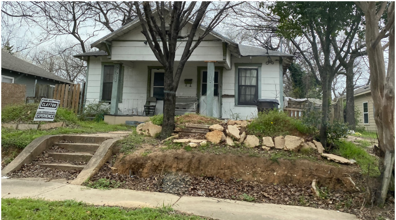
Figure 17 Street view of South Dallas Neighborhood -Abandoned property
