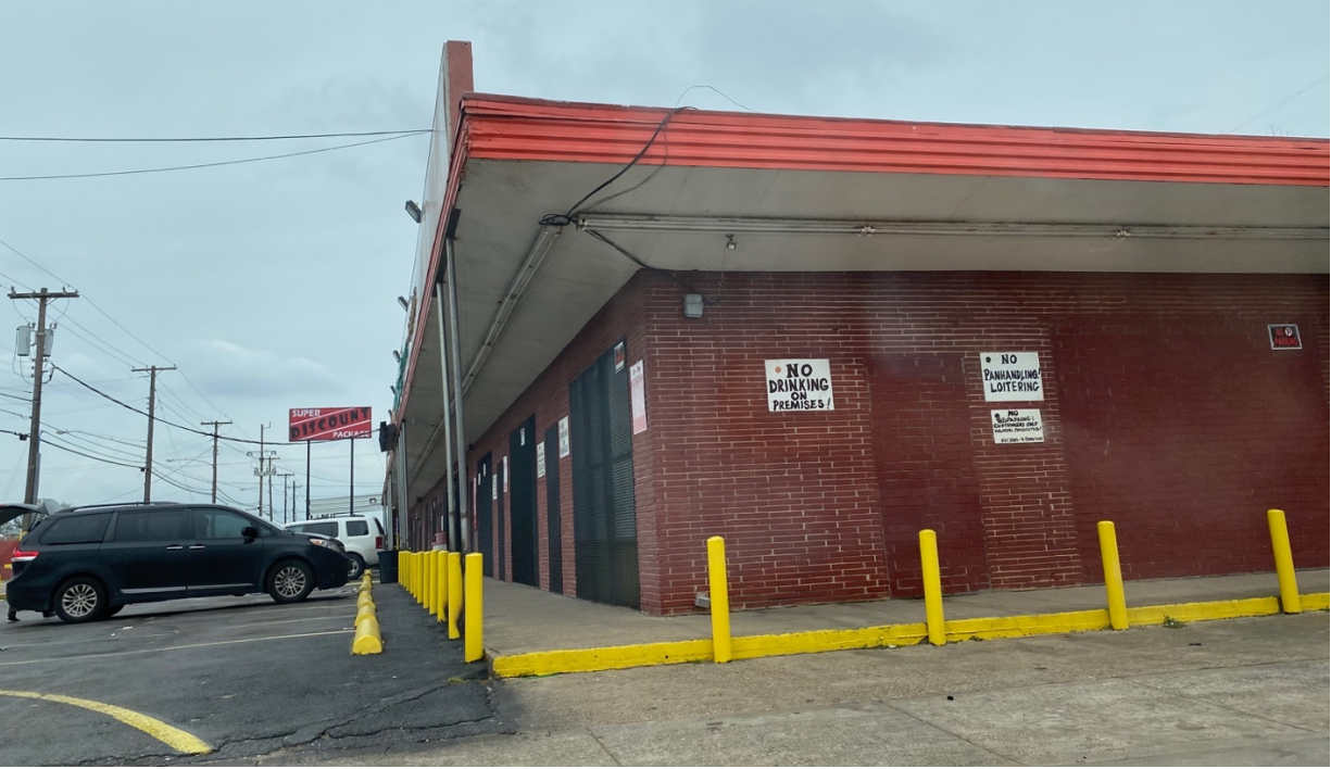
Figure 24 Street view of South Dallas Neighborhood – signs of no drinking and no loitering
