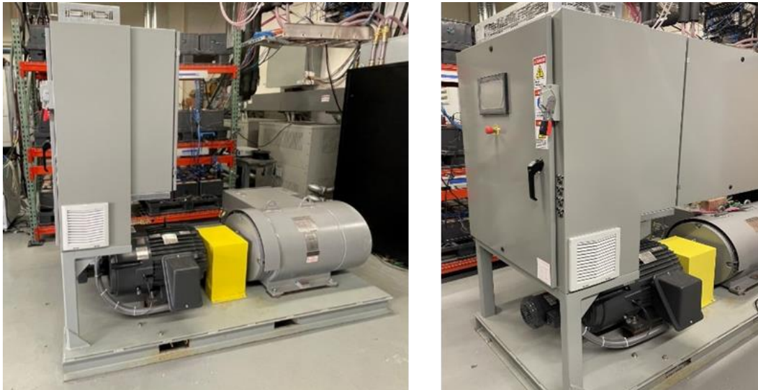
Figure 50. Photographs showing the 40-kW machine after installation.
