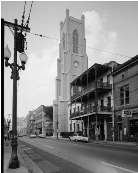
Figure 8. James Gallier and James Dakin, St. Patrick's Church, Camp Street, 1838–40. Dan Leyrer, photographer, September 1963. Source: Historic American Buildings Survey, HABS LA, 36-NEWOR, 59-1.
