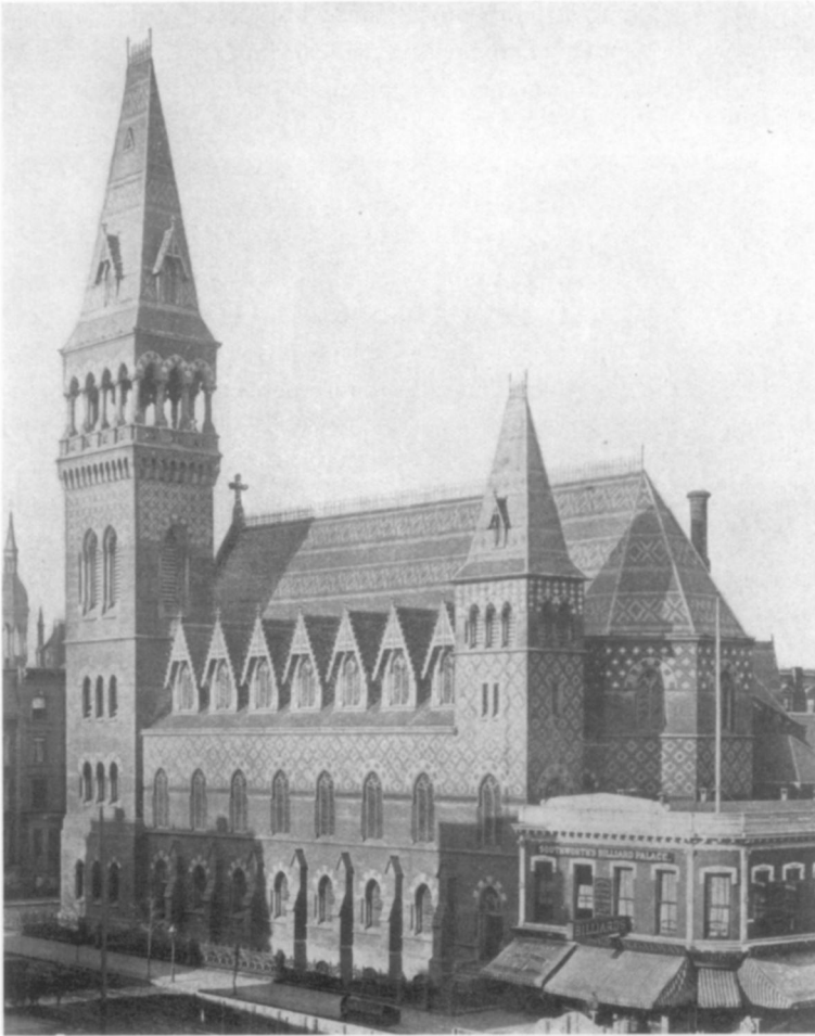
Figure 3 Leopold Eidlitz, Church of the Holy Trinity, New York, corner of Madison Avenue and 42nd Street, 1873–74. Demolished
