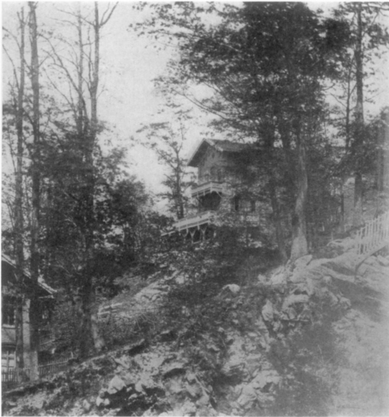
Figure 7 Leopold Eidlitz, Eidlitz Residence, New York, 1851. At present-day Riverside Drive and 86th Street. Demolished
