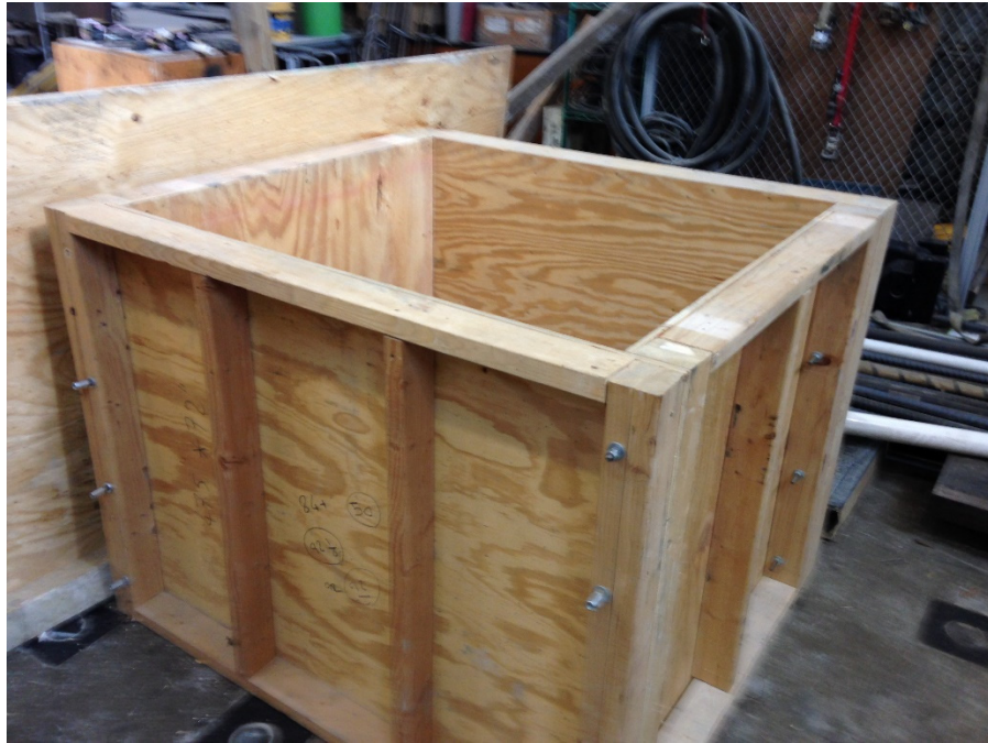
Figure 3- 10 The formworks of the concrete block that supports the actuator.
