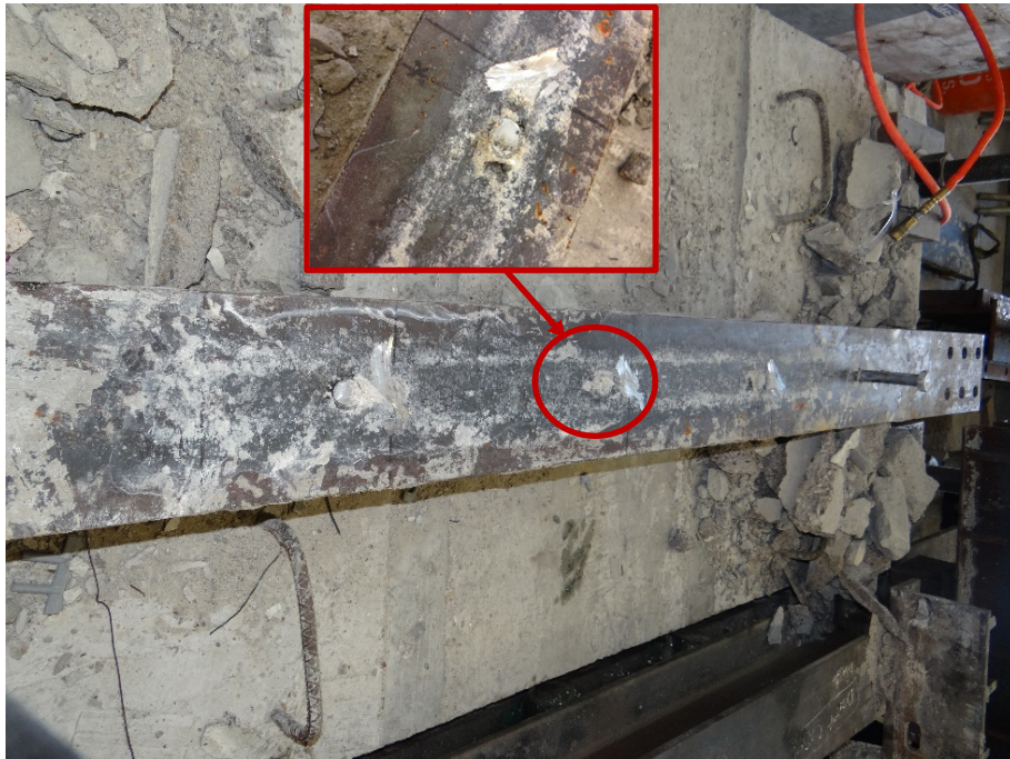
Figure 4-42 Fractured section of the shear stud after failure at (+57 Kips).
