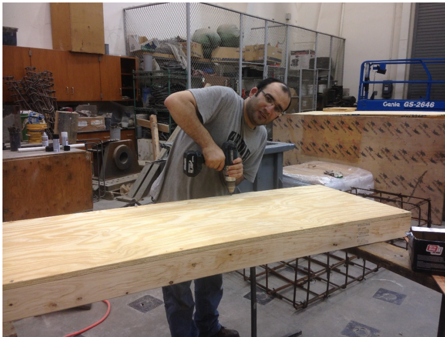
Figure 3-7 Preparing the sides of the formworks.
