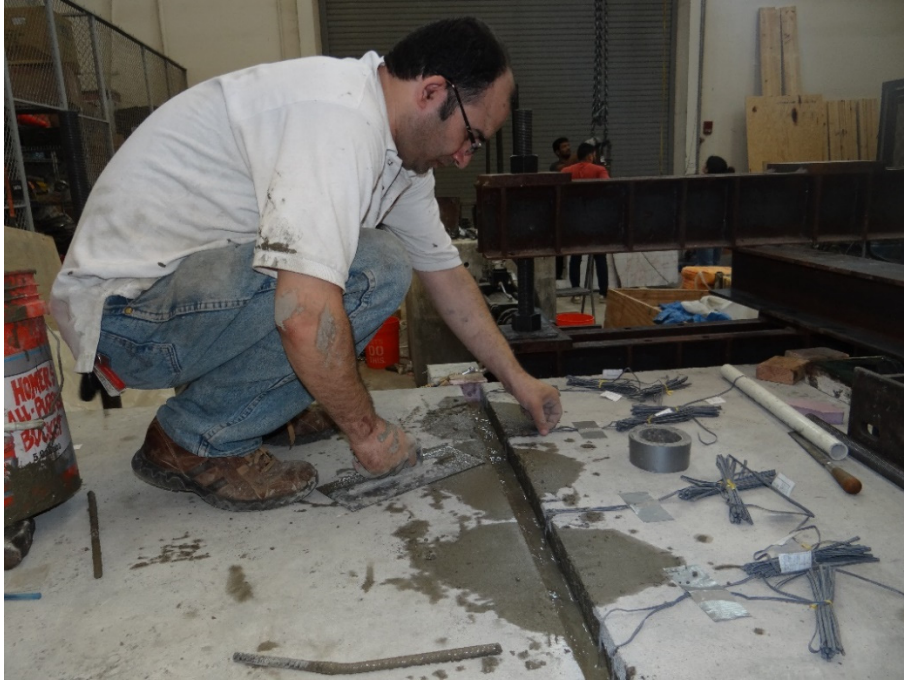
Figure 3-38 Filling the connection and the holes in the planks.
