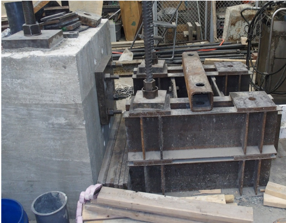
Figure 3- 42 Supporting the actuator's concrete block from the back.
