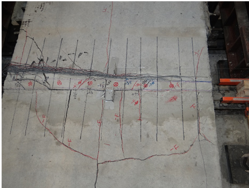
Figure 4-80 Overview of the cracks at -55 Kips.
