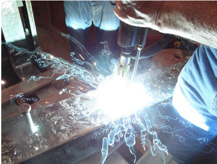
Figure 3-26 Melting the welding stud base and the area of the steel beam and escaping the weld gases through vents in the ceramic ferrule.
