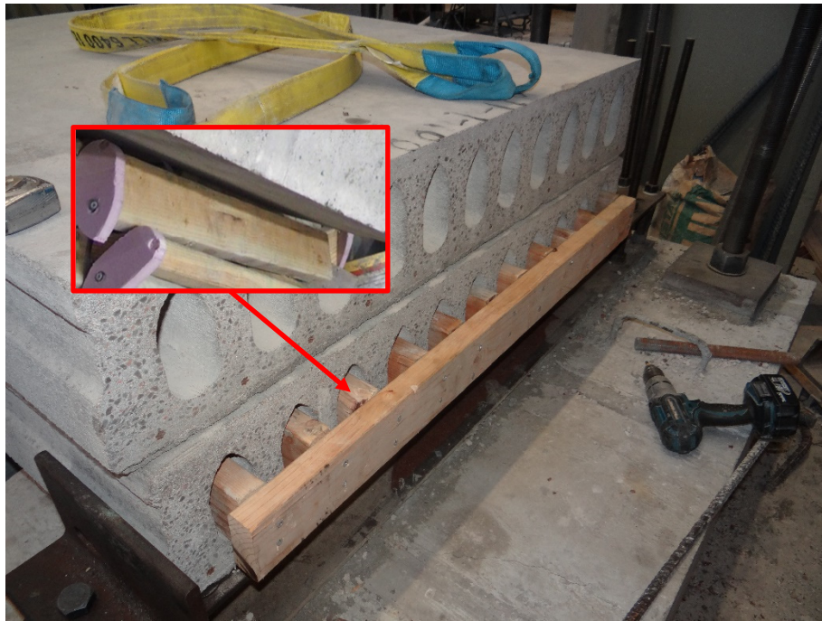
Figure 3-35 Closing the holes in the planks at the ends of rebars.
