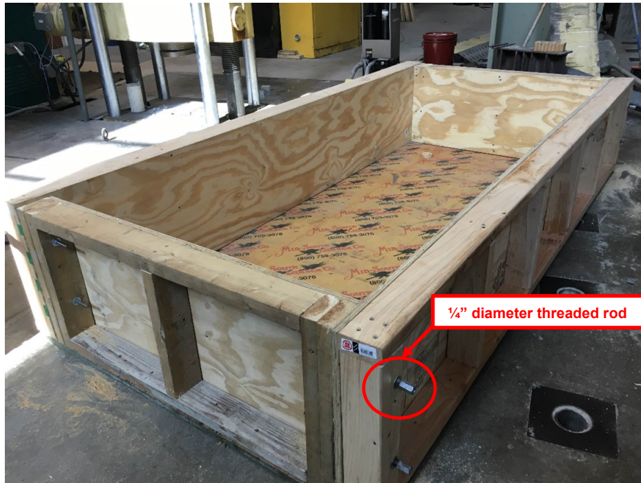
Figure 3-8 Connection the sides of the formwork together.
