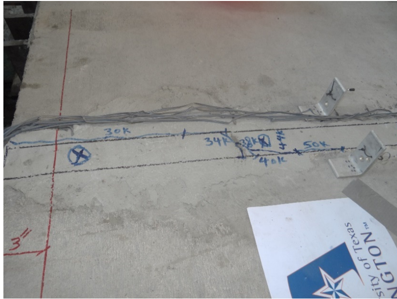
Figure 4-6 Crack propagation in the fixed side at 50 Kips.
