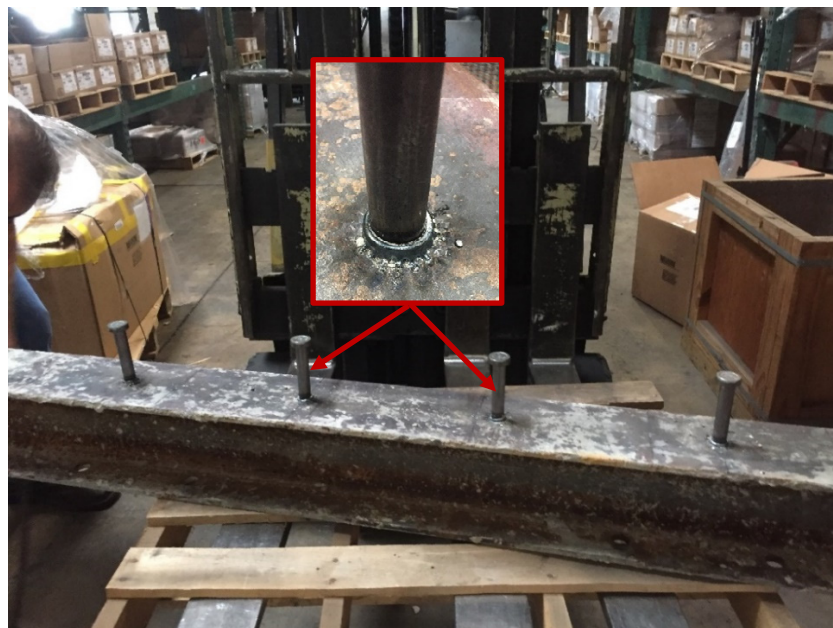
Figure 3-27 The shear studs and the welding area (in the frame) after completion of the welding process.
