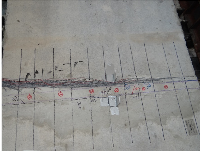
Figure 4-78 Diagonal cracks also at -50 Kips.
