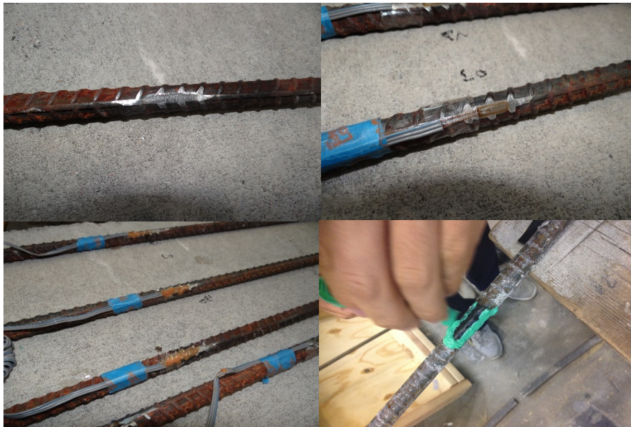
Figure 3-53 Strain gauges installing process on the longitudinal rebars.
