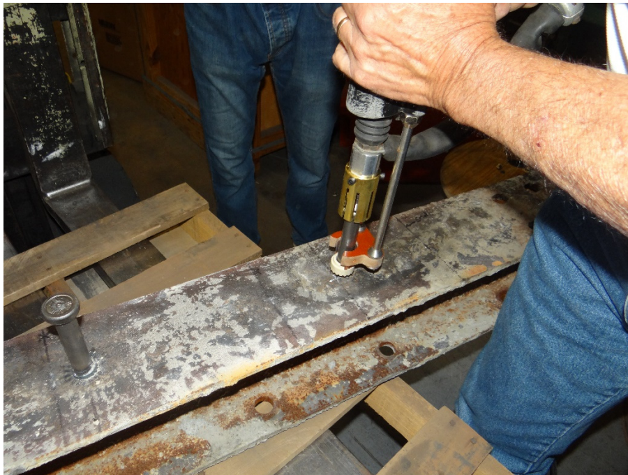
Figure 3-25 Placing the shear stud in contact with the steel beam
