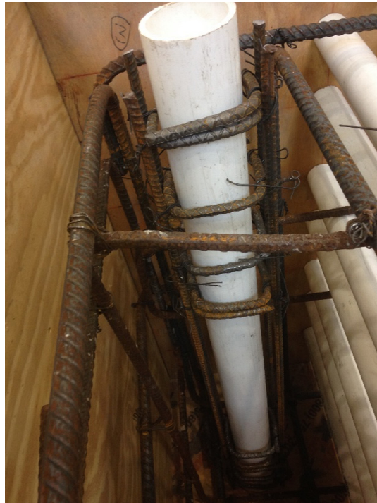
Figure 3-13 Stirrups at the ends of the PVC pipes.
