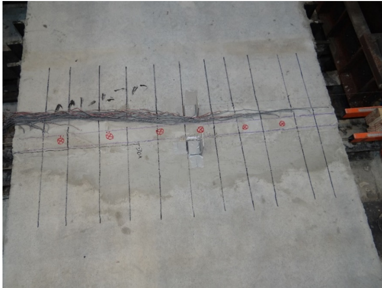
Figure 4-71 The first crack in the connection (at +30 Kips) for cyclic in-plane shear deformation (6 Studs, 180° hooked rebars) test.
