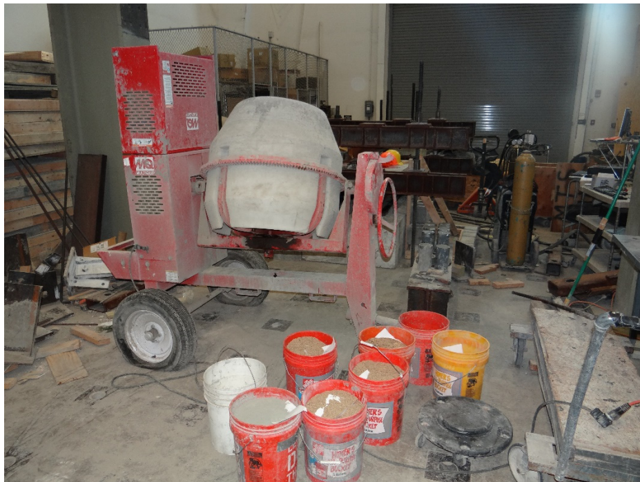
Figure 3-37 Preparing the materials for casting the connection.
