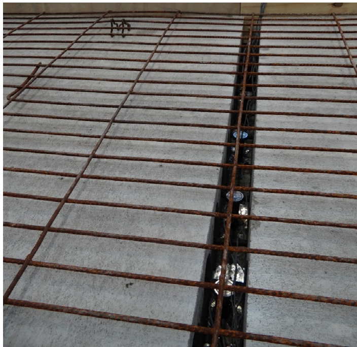
Figure 3-65 Steel reinforcement mesh of the concrete topping slab over the connection.
