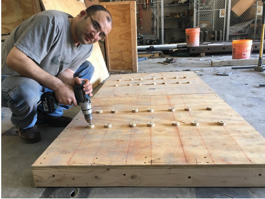
Figure 3-12 Installing the plywood discs to support the PVC pipes.
