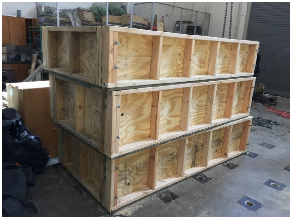
Figure 3-9 The formworks of the three concrete blocks that support steel beams.
