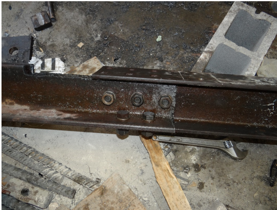
Figure 3-45 Connecting the W6X25 steel beam to the two steel angles.
