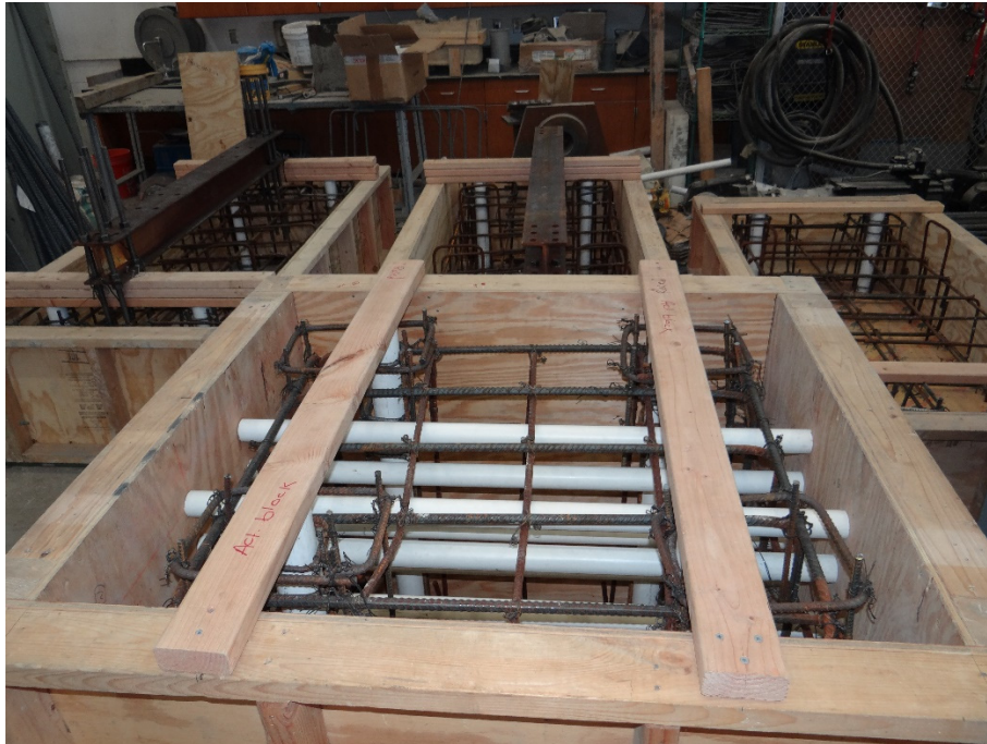
Figure 3-16 Complete specimens' components before concrete casting.
