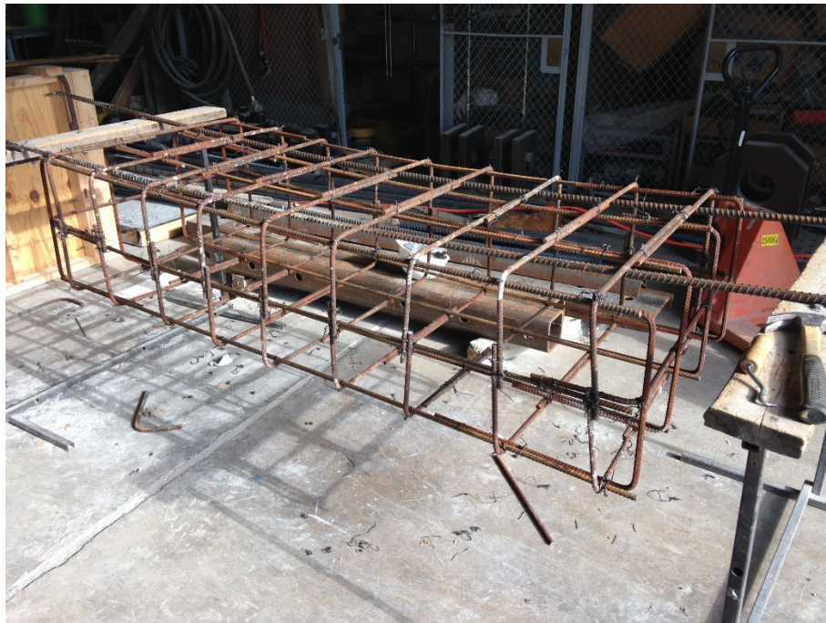
Figure 3-11 Preparing the steel cages.
