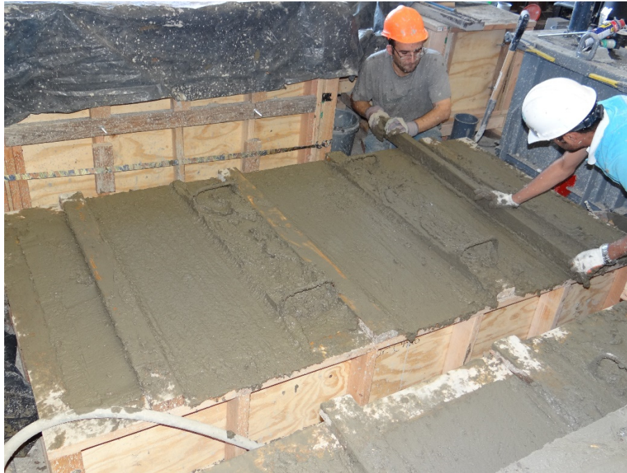
Figure 3-18 Finishing the surface of the specimens after casting.
