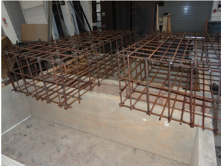
Figure 3-75 steel cages reinforcement and the formworks of the blocks.
