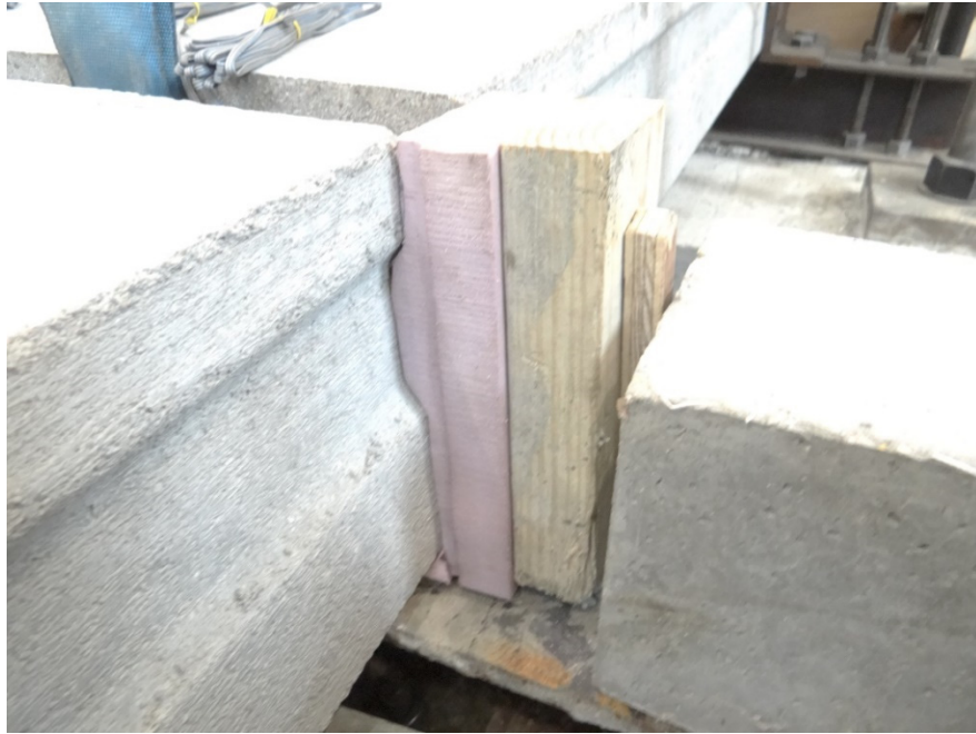
Figure 3-36 Closing the ends of the connection.
