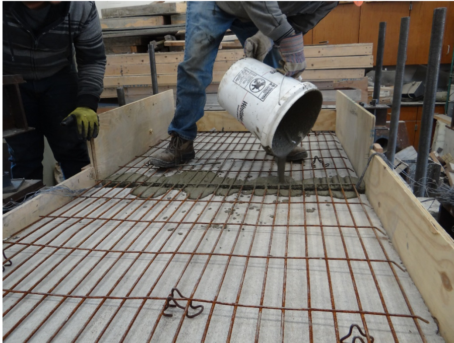
Figure 3-66 Casting the connection first then the concrete topping slab.
