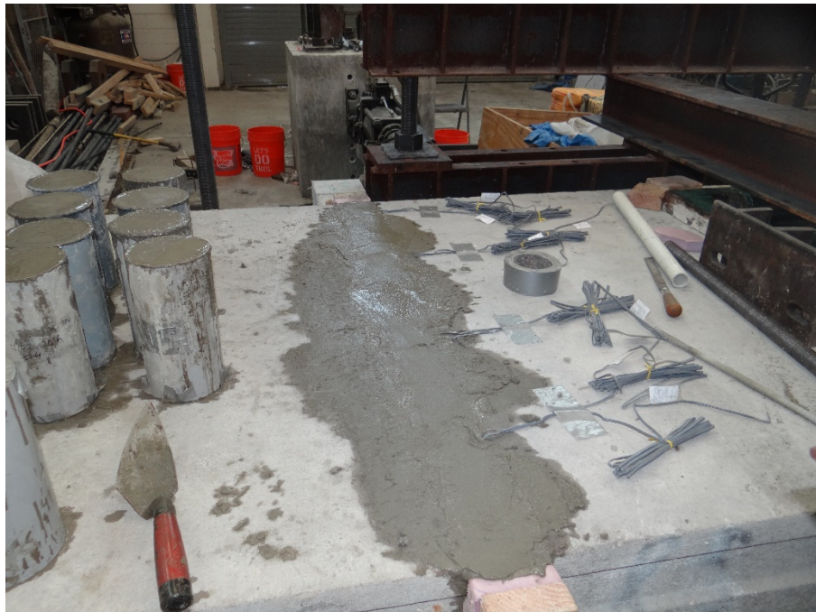
Figure 3-39 The connection after completion the casting.
