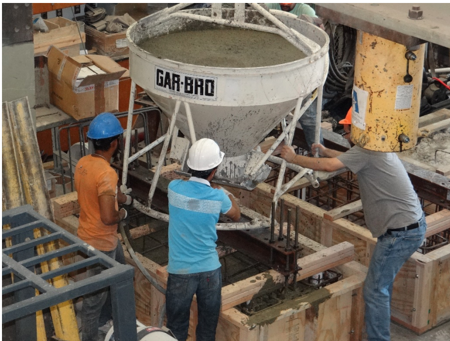
Figure 3-17 Concrete casting of the specimens.
