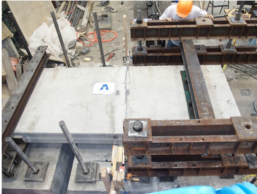
Figure 3-51 Top view of the setup before testing the specimen.
