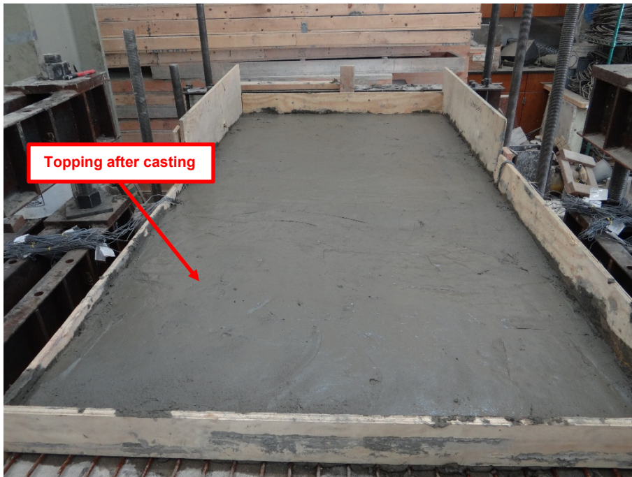
Figure 3-67 The concrete topping slab after completion casting.
