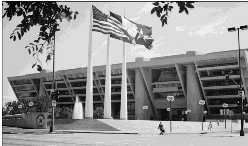
Figure 4-4. The Dallas City Hall, Dallas, Texas
