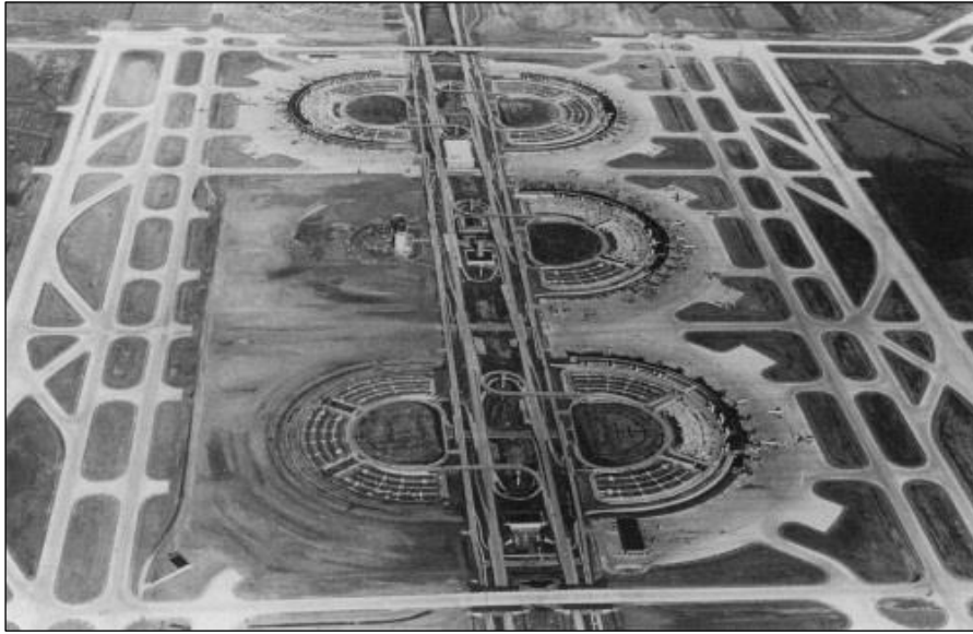
Figure 4-5. DFW Airport during construction in 1973
