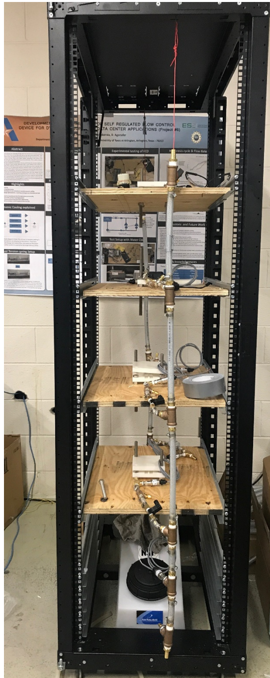
Figure 0-2 Experimental setup in progress for Control Strategy Validation
