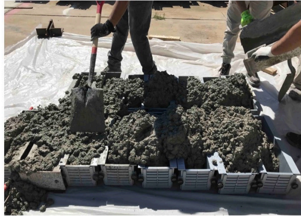
(b) spreading the concrete into the mold
