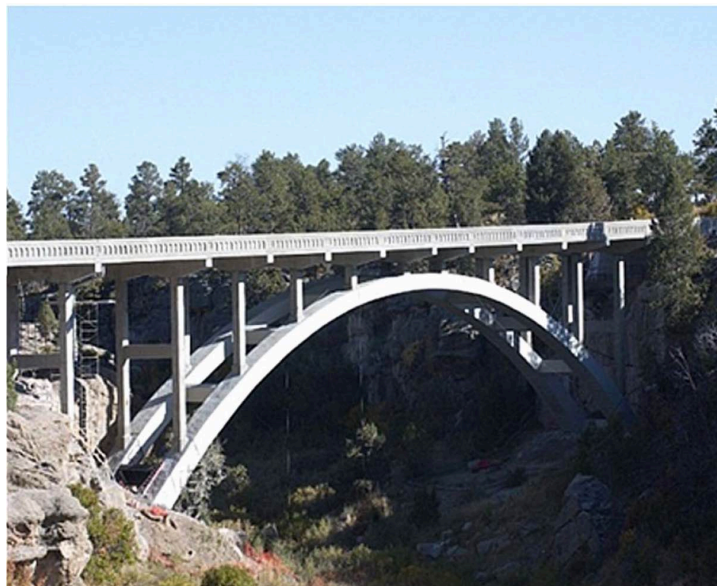
Figure 2-6 Castlewood Canyon Bridge (Allen and Atadero, 2012)
