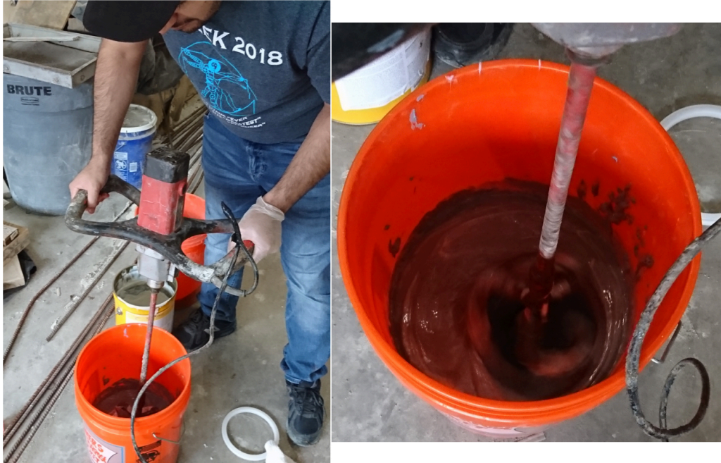
Figure 3-2 Mixing the two-part epoxy resin
