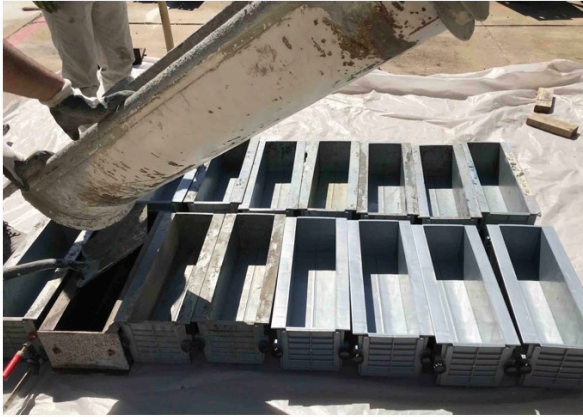
(a) pouring the concrete into the beam molds
