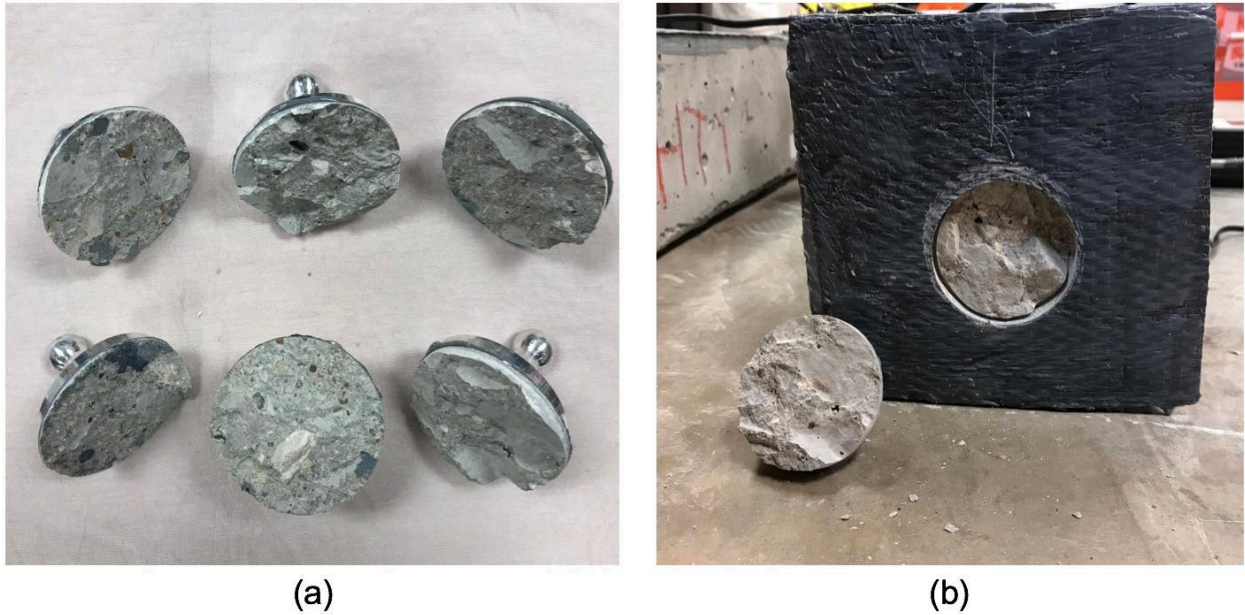
Figure 4-17 (a) various observed failure modes, (b) dolly next to its original location
