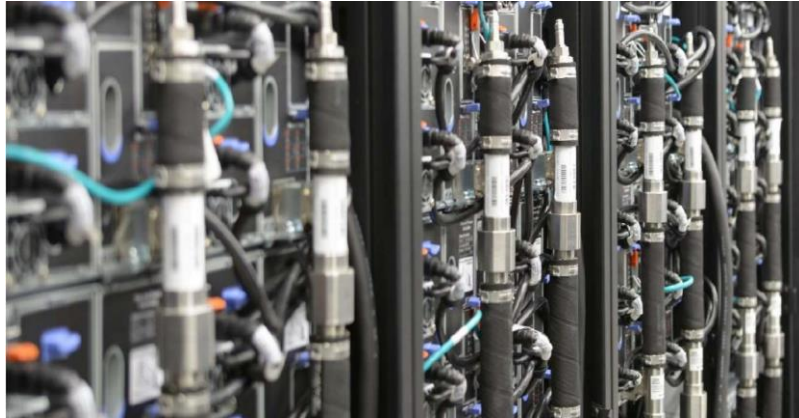
Figure 7: piping of liquid cold plate[7]
