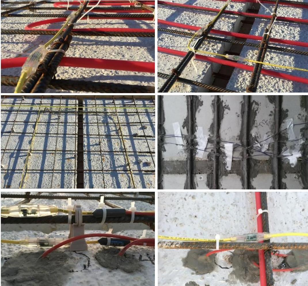
Figure 3.10. Stage 3 of the fieldwork: Bridge deck instrumentation
