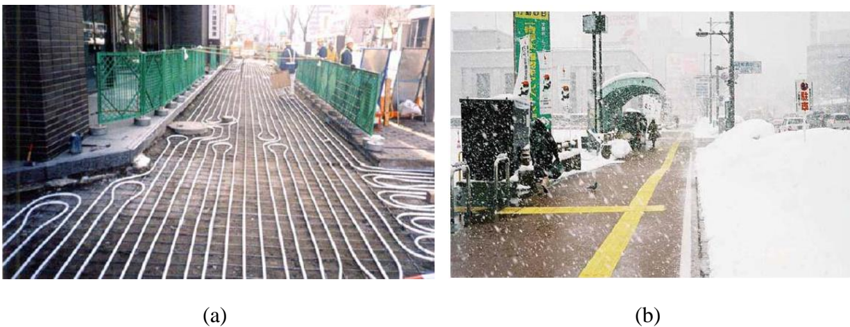
Figure 2.7. Sidewalk snow-melting project in Aomori, Japan: (a) Hydronic heating loop; (b) System under operation (Morita and Tago 2005)
