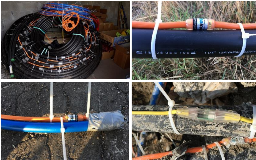
Figure 3.16. Subsurface soil and underground loop instrumentation
