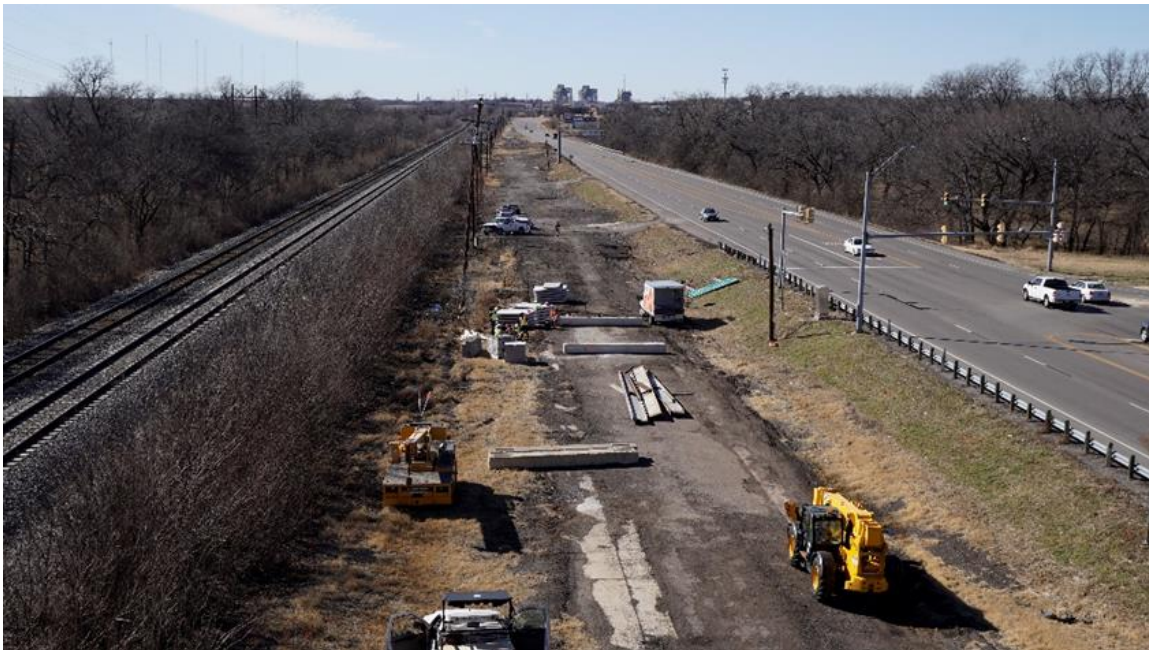
Figure 3.1. Photo of the construction site located in Fort Worth, TX
