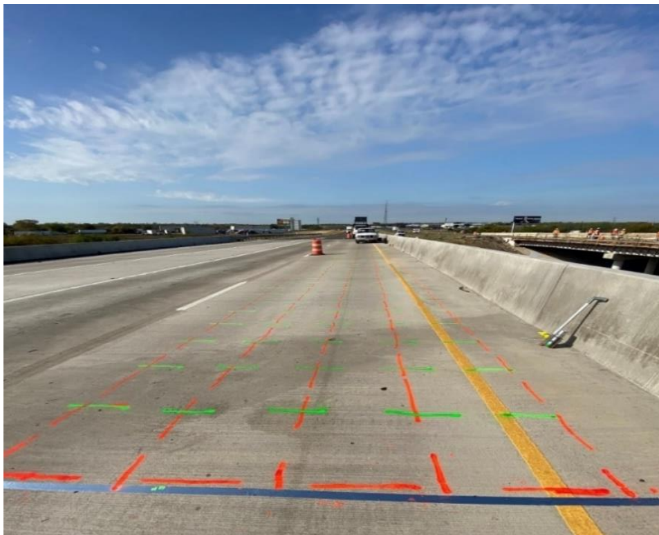
Figure 4-19: GPR and IE scanning grids
