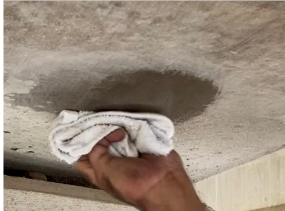
(b) Cleaning surface with acetone
