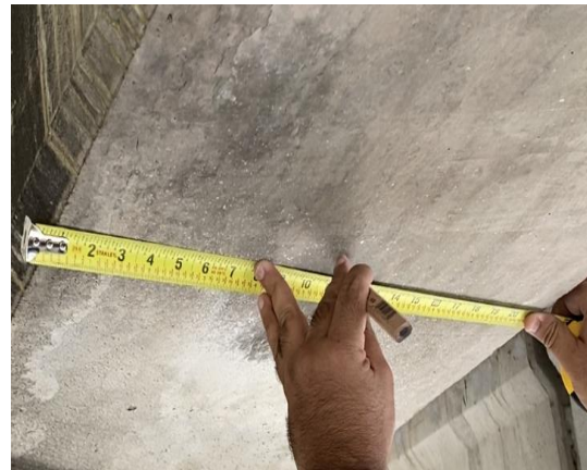
(d) Measuring mid-point of girder
