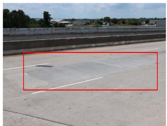
Figure 1-5 Failure patterns in span 2 of EB bridge (TxDOT): (a) CIP deck; (b) PCPs
