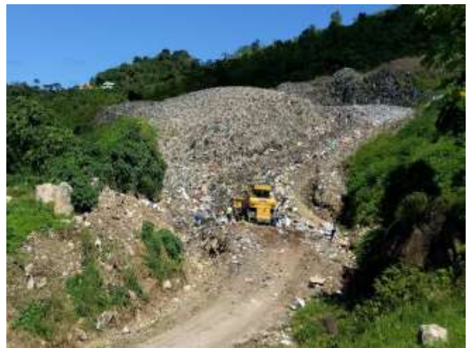
Figure 2.7. Track loader operation
