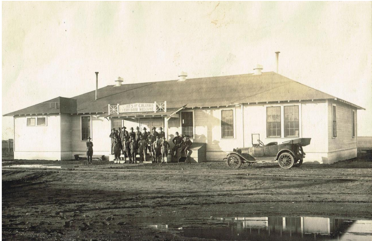
Figure 21. Knights of Columbus Hall, Call Aviation Field, Wichita Falls, Texas, ca. 1918. Photo courtesy of the Museum of North Texas History, Wichita Falls, Texas.
