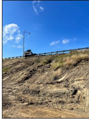
Figure 5.17 Backfill of Slope.
