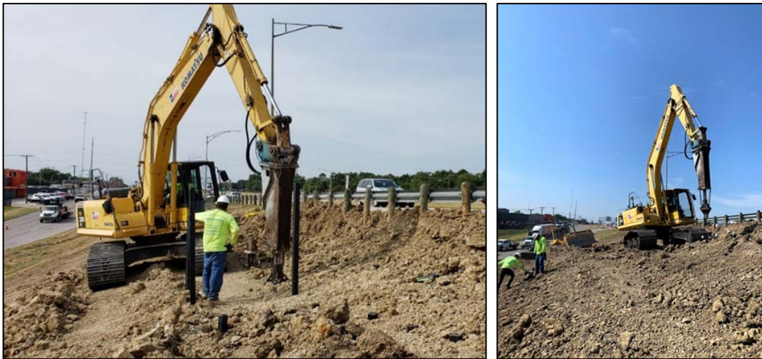
Figure 4.11 Installation of Deeper Pins.
