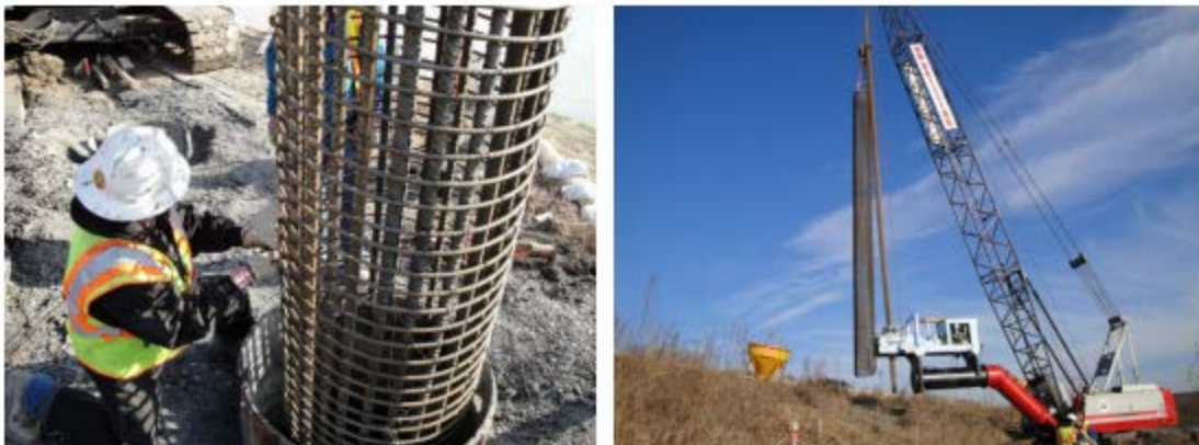
Figure 2.13 Construction of Drilled Shafts.
