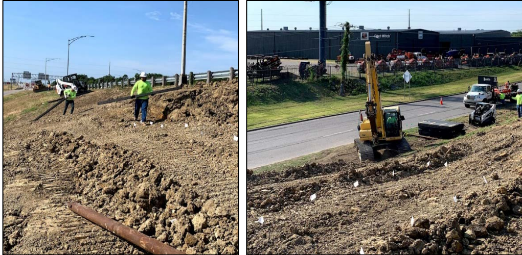
Figure 4.10 Benching and Compaction of the Crest of the Slope.
