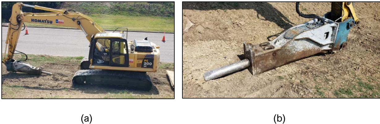
Figure 4.9 RPP Installation Equipment; Excavator Equipped with Hydraulic Hammer, (b) Hydraulic Hammer
