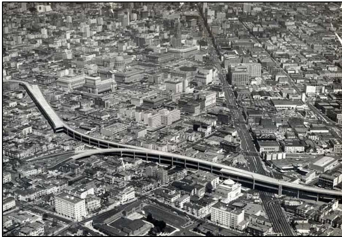
Figure 13 – Central Freeway Source: sfgate.com
