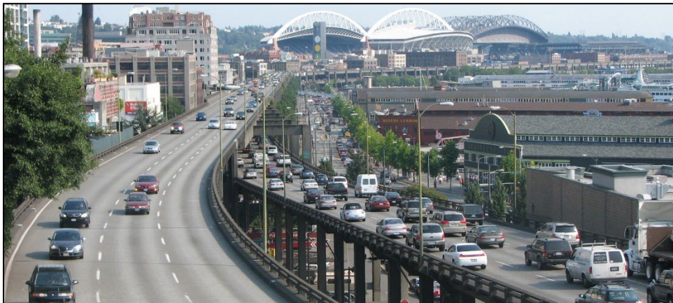
Figure 18 – Alaskan Way Viaduct Source: cnu.org
