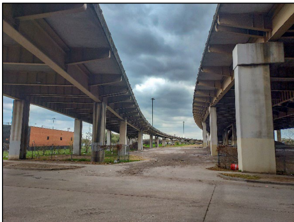
Figure 32 – Vacant Land Under I-345
