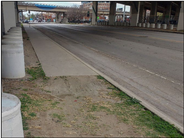
Figure 27 – Sidewalk Dead Ends Abruptly Under I-345
