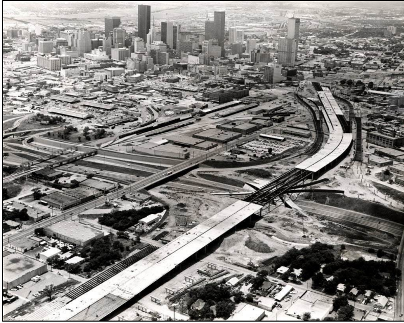
Figure 1 - I-345 Under Construction in Early 1970s Source: aiadallas.org
