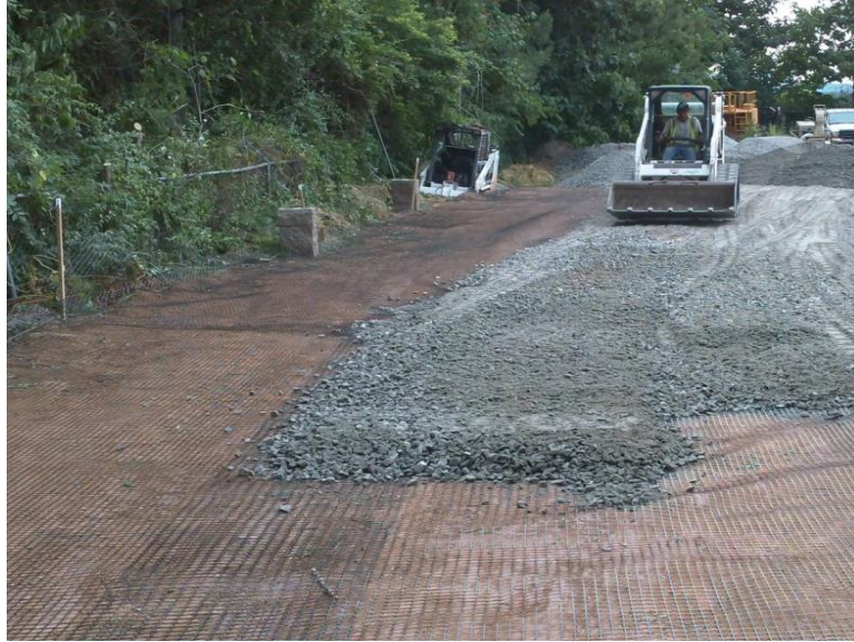
Figure 2-8 Use of geo-grid for subgrade treatment
