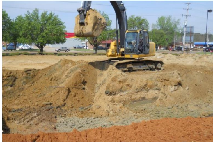
Figure 2-6 Removal of soil for subgrade treatment
