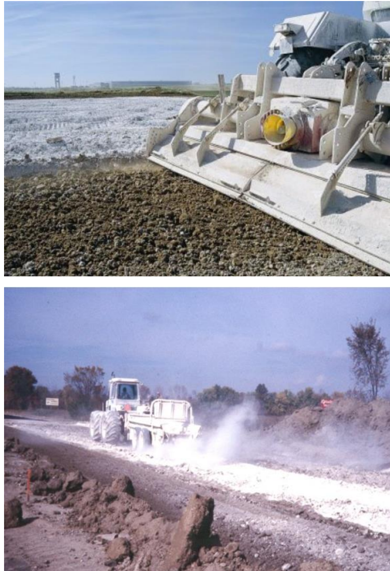
Figure 2-9 Mixing additives for subgrade treatment
