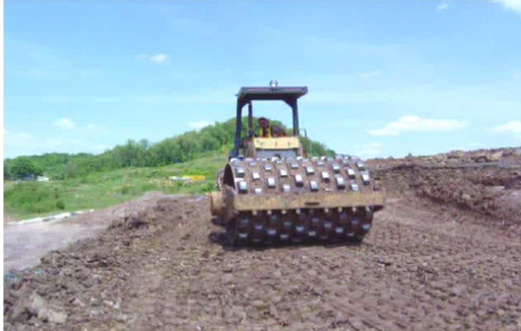
Figure 2-7 Traditional compaction method for subgrade treatment
