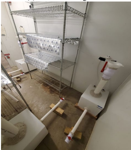
(c) Anaerobic Digester 3
