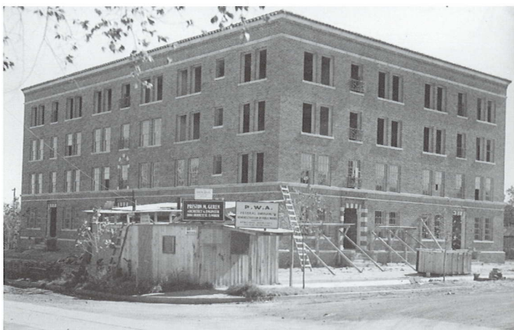
5.11 Davis Hall, now known as Brazos House, was completed in 1936 with federal funding through the Public Works Administration. According to the 1937 Junior Aggie , a student described it this way: “Remember splintered feet, cold showers, shaving rushes, freezing mornings, blown fuses—they days are gone forever, we’re living in a real Ho-tel!”
