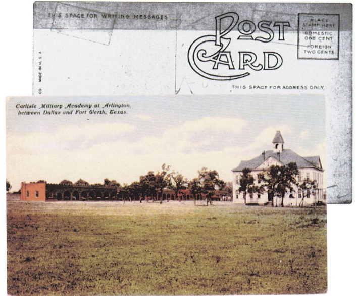
2.8 Described as a fireproof, modern brick building with concrete floors, the East Barracks, pictured on this post card, served as the men's dormitory. Having designed the dormitory's folding iron beds himself, Carlisle called them "the best student beds in use, being free from bugs, and convenient."
