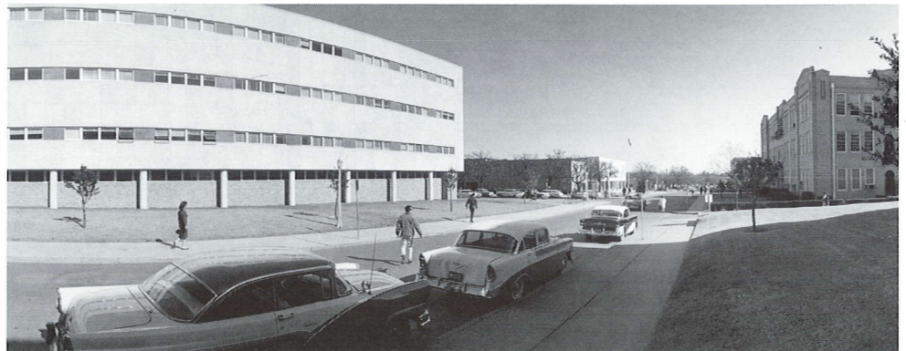
6.16 When the Engineering Building was built on the old college parade grounds in 1960, it not only enjoyed the distinction of being the largest classroom building in the Texas A&M system, but also completed the present configuration of buildings along Second Street.
