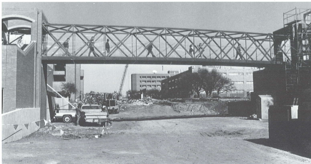
7.32 Noted as a hazard as early as the mid-1960s, the Cooper Street crossing problem was finally solved in 1990, when the street was partially depressed and three walkways were constructed over it.
