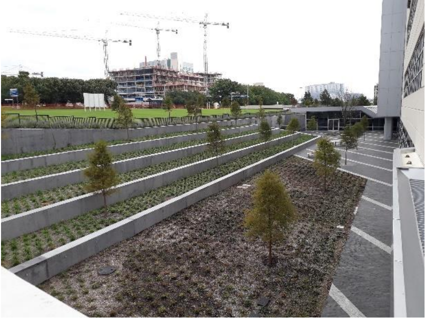
A Garden That Provides Light and View for the Restaurant and Kitchen of the Hospital
