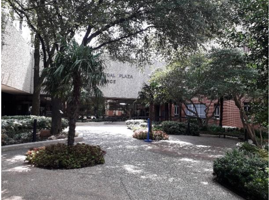
Baylor Medical Plaza Entrance with Transparent Walls and Views to Plaza Garden
