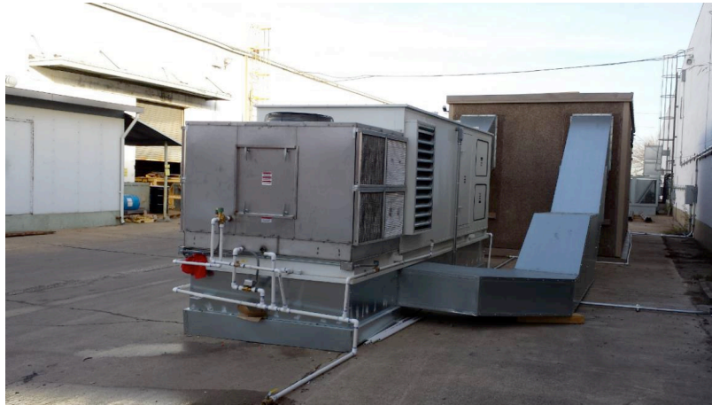
Figure 6: Return Duct Arrangement of MDC [15]
