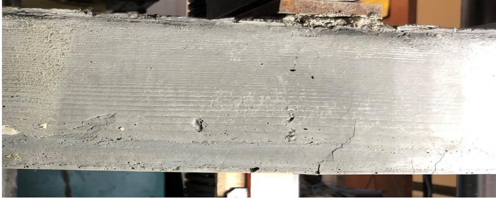
Figure 3-9 Cracking of specimen 3#3: a) initiation, b) at the end of the test c) shear cracking
