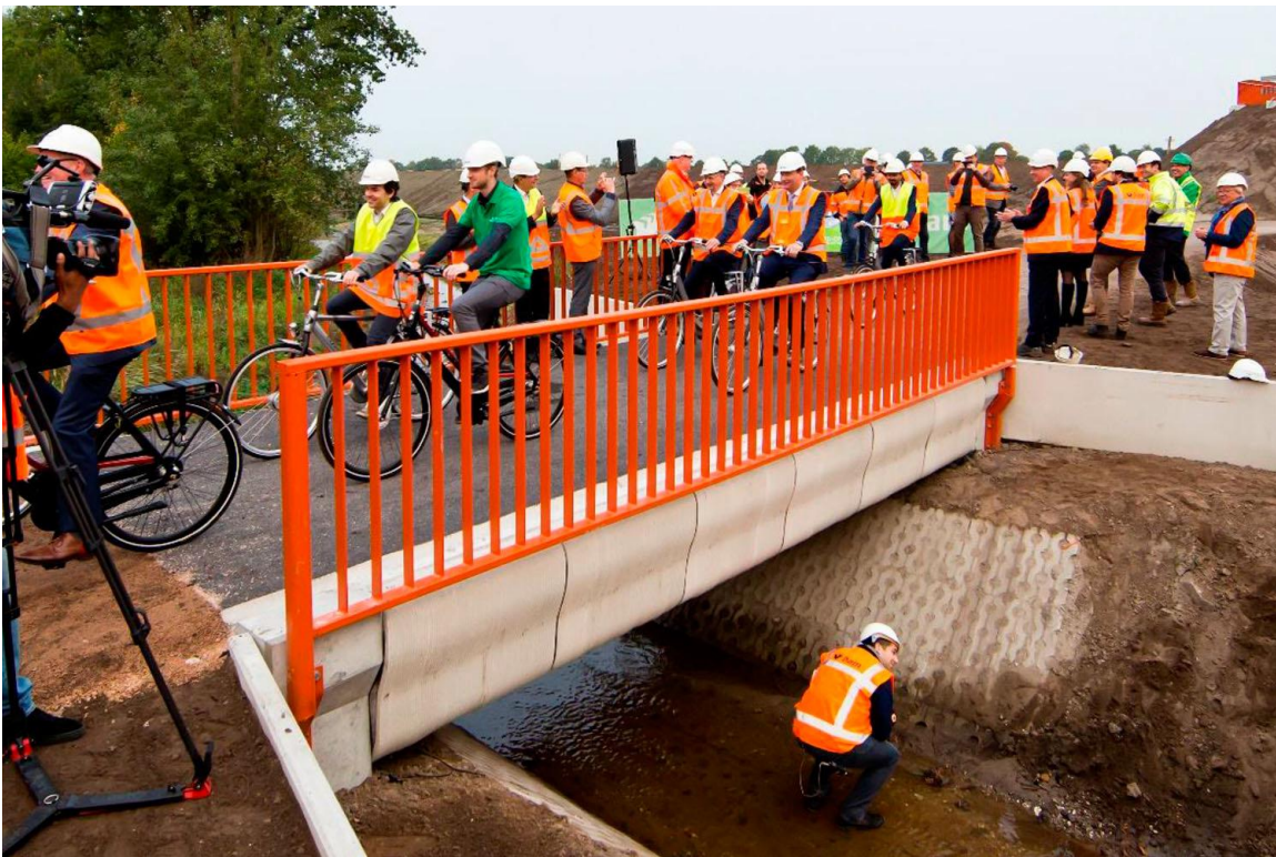
Figure 2. 1 3D Printed Concrete Bridge (Salet et al., 2018)
