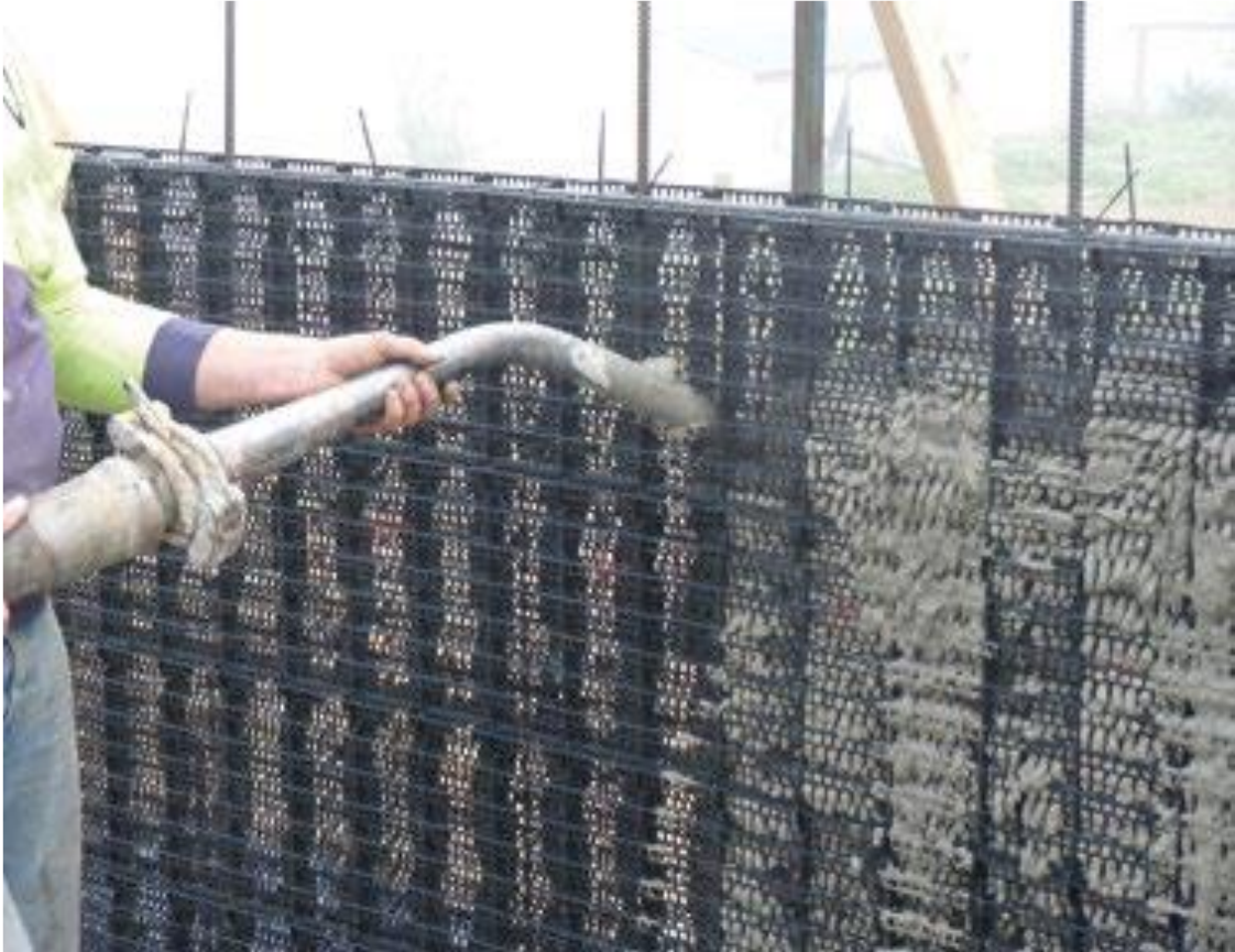
Figure 2. 4 Mesh Mould Technique of Reinforcement in Digital Fabrication (Hack et al., 2015)
