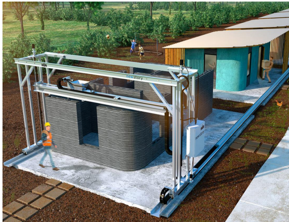
Figure 1. 1 3D Printed House (contour crafting)
