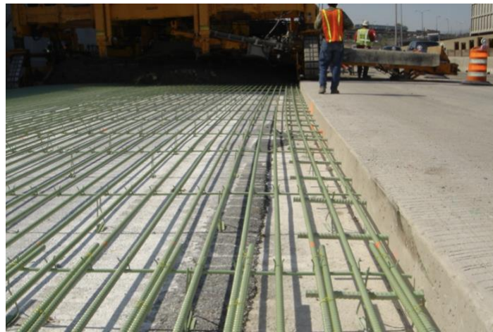
Figure 2-7. reinforcement steels in continuous reinforced concrete pavement.
