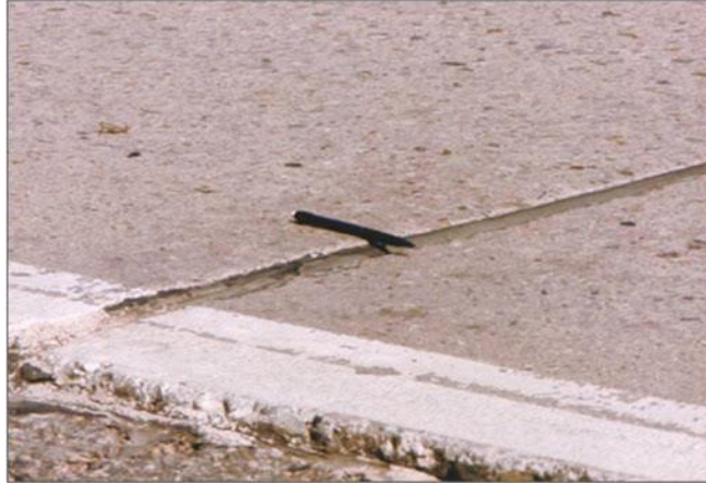
Figure 2-9. Joint faulting
