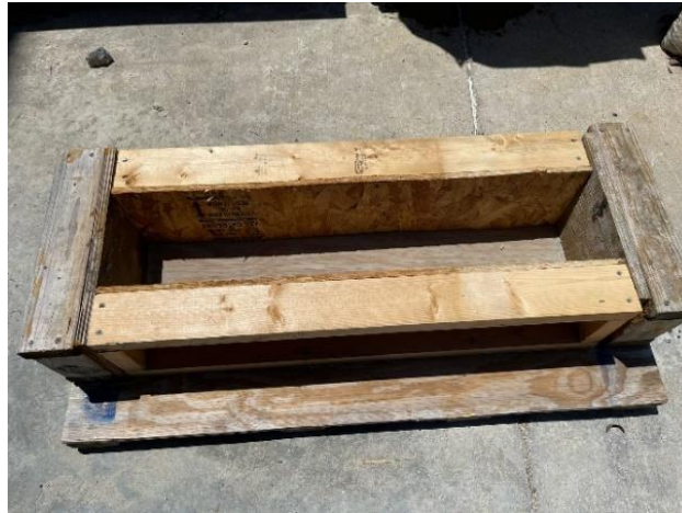
Figure 17: Beam formwork
