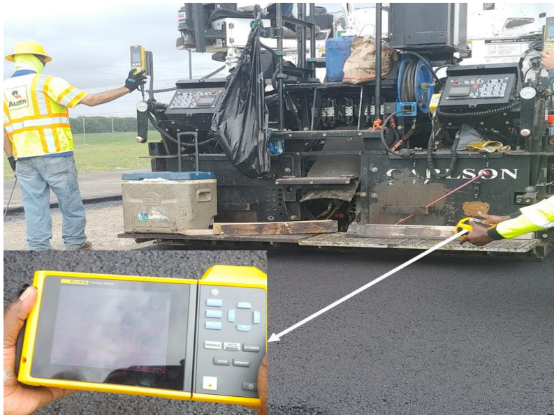
Figure 3.26 The Infra-Red Camera Recording Pavement Construction Temperature
