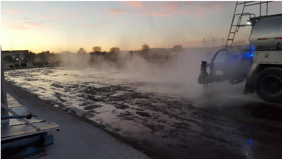
Figure 3.16 Spraying of Prime Coat on top of the flex base
