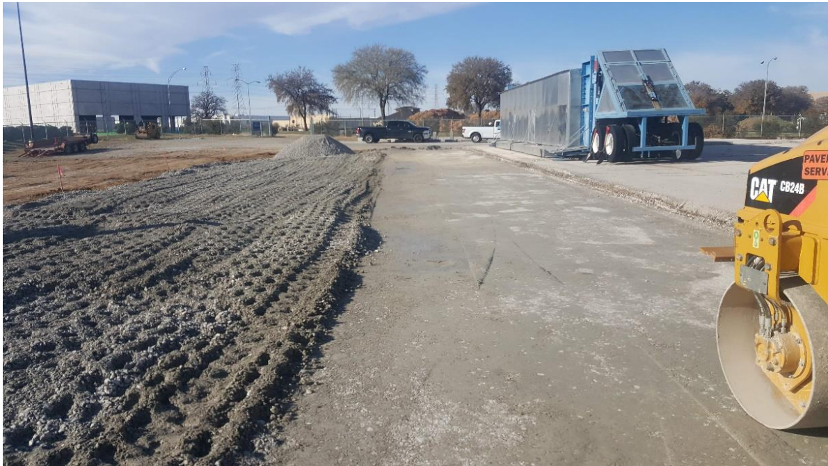
Figure 3.14 Compaction of flex base -top lift
