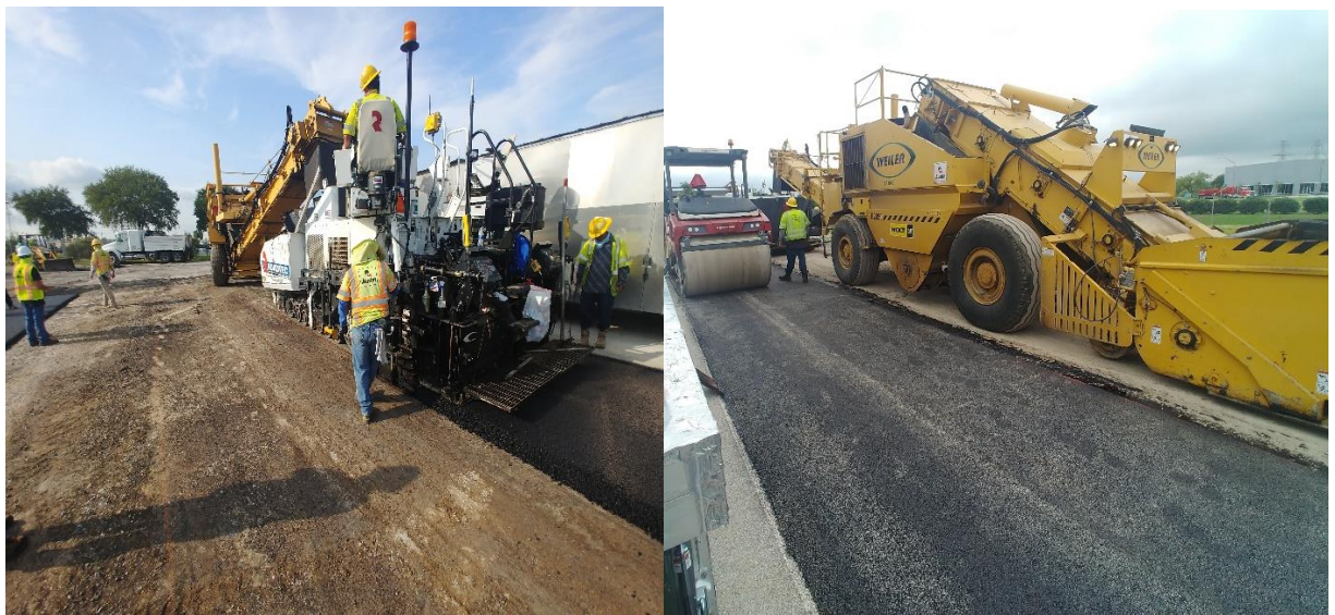
Figure A4-2 Paving of sections M and Q (same mixtures for two sections)
