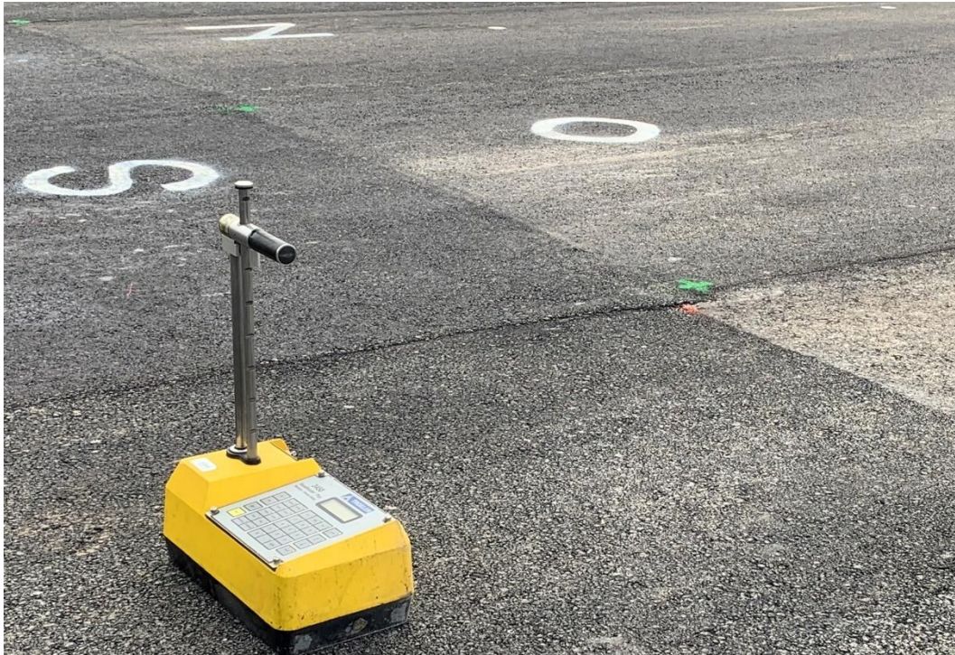
Figure 3.28 Measuring Field Density Using the Nuclear Density Gauge
