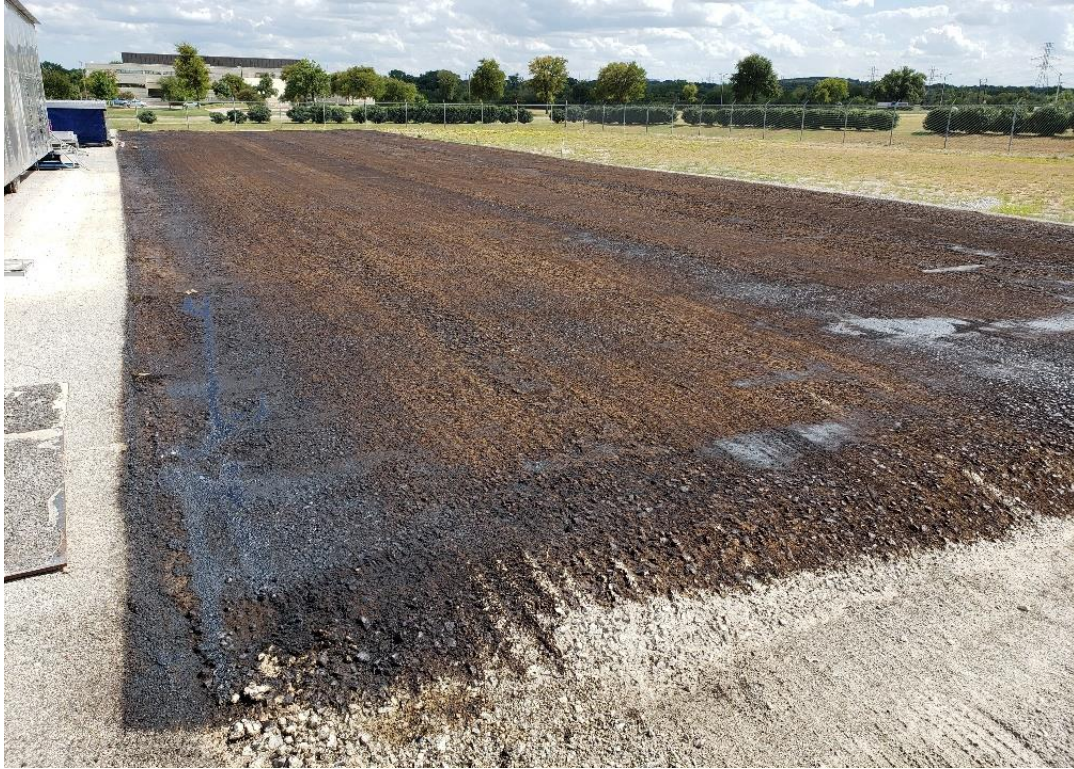
Figure 3.17 Constructed base layer with Prime coat
