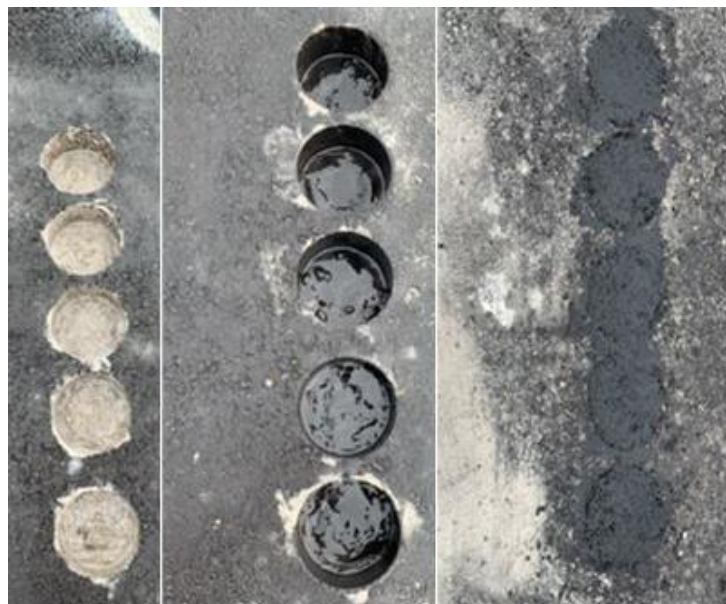
Figure 4.2 Sequence of covering the core holes
