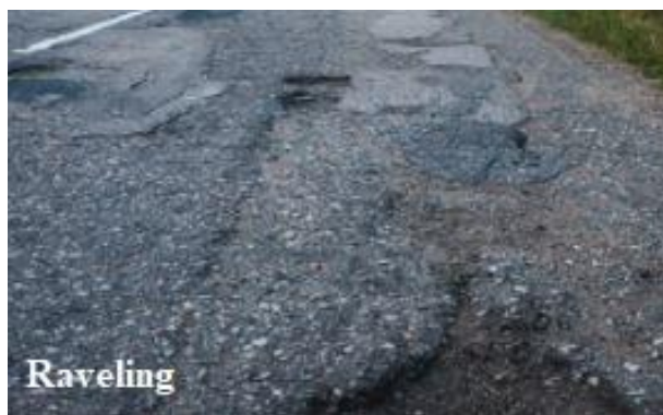
Figure 2.12 The most predominant asphalt distresses across United States (NCAT, 2017)
