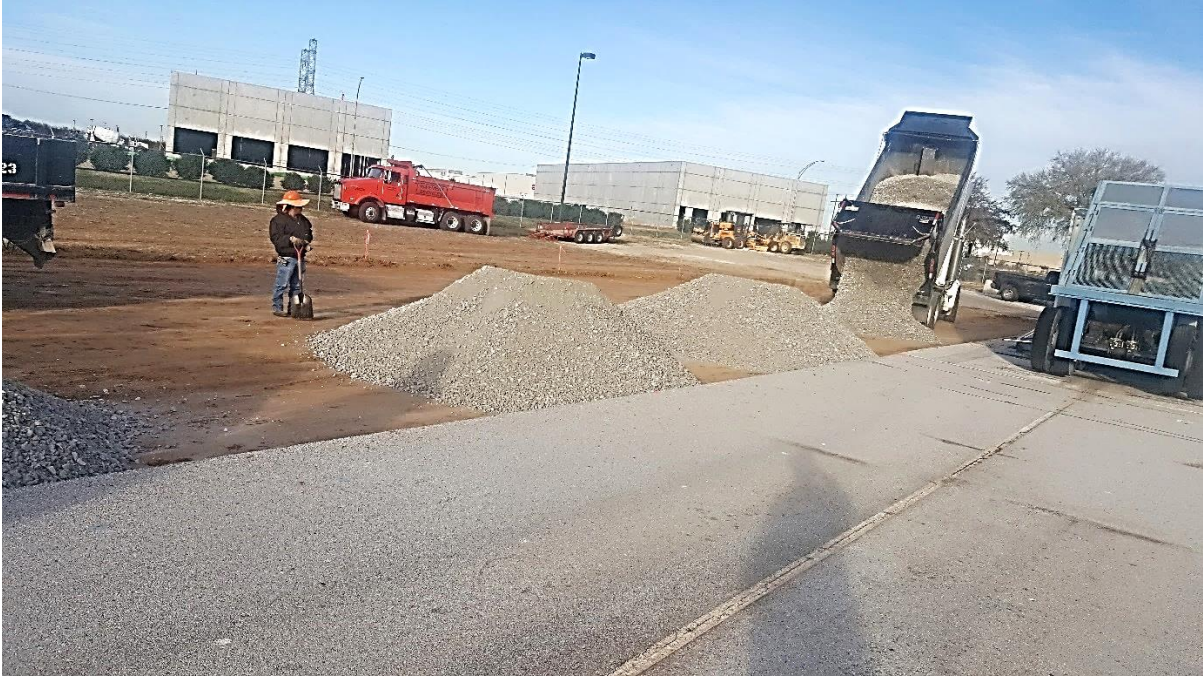
Figure 3.13 Placement of flex base
