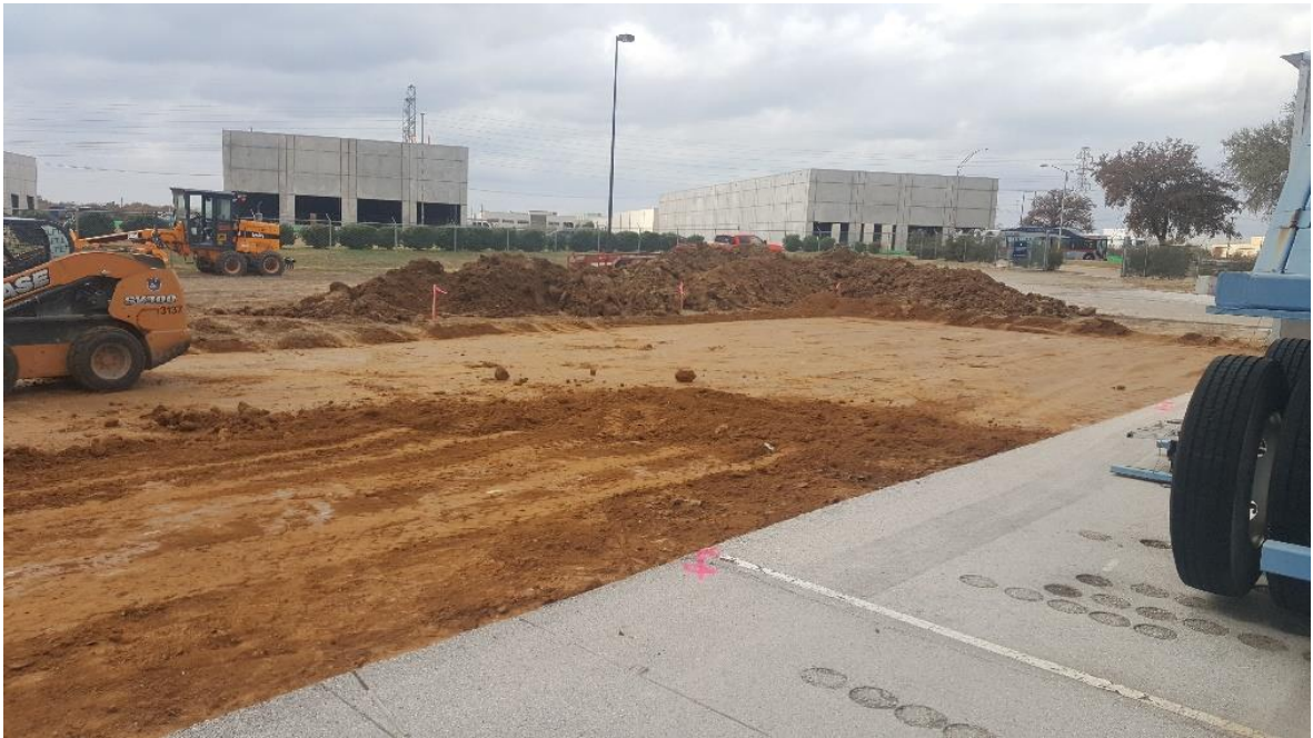
Figure 3.9 Placement of new subgrade soil
