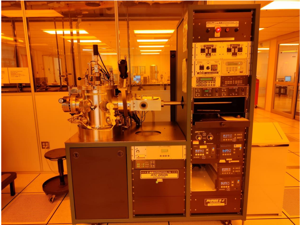
Figure 27: AJA Sputter Deposition equipment for DC and RF Sputtering
