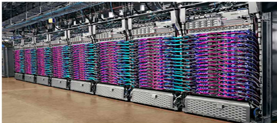
Fig 1: liquid-cooled 1U rack data center[3]
