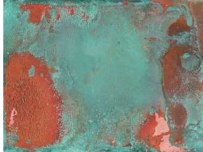
Fig 5: corroded copper surface
