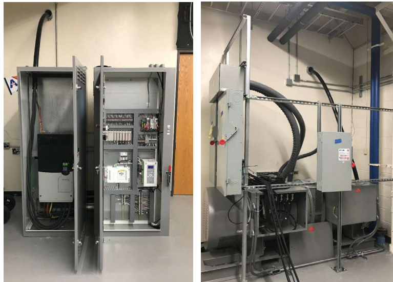
Figure 1.4: Photographs showing the M-G set (left) and internals of the control and VFD cabinets (right).
