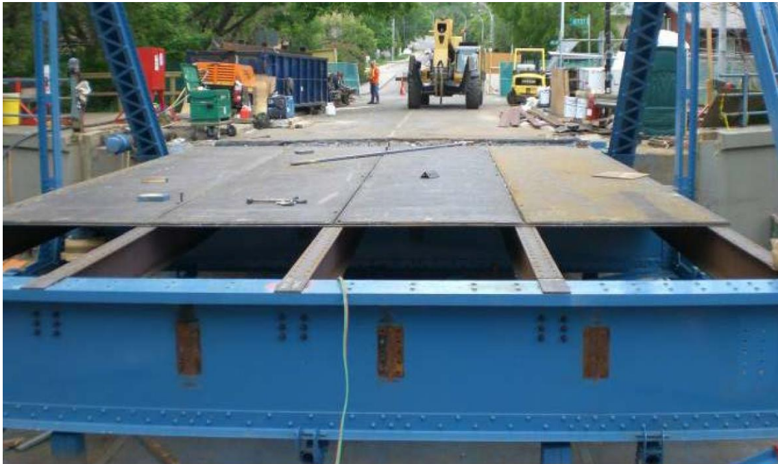
Figure 2- 15 Re-decking of Dawson Bridge (Dialog 2010)
