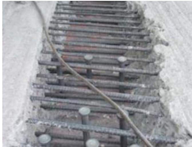
Figure 2- 21 Welded headed studs welded to the steel girder (Collin et al. 2015)
