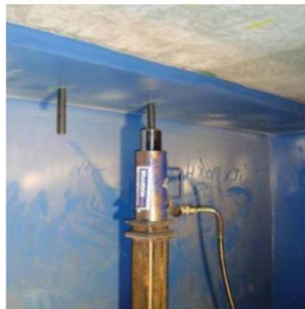
Figure 2- 26 Hydraulic jack used for inserting spiral pins into the bridge (Collin et al. 2015)
