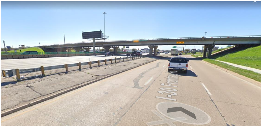
Figure 3- 2 Bridge side view (Google Earth)
