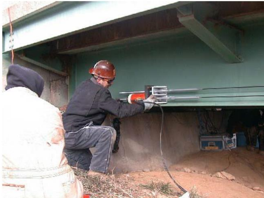
Figure 2- 17 Installation of PT system (Terry et al. 2003)
