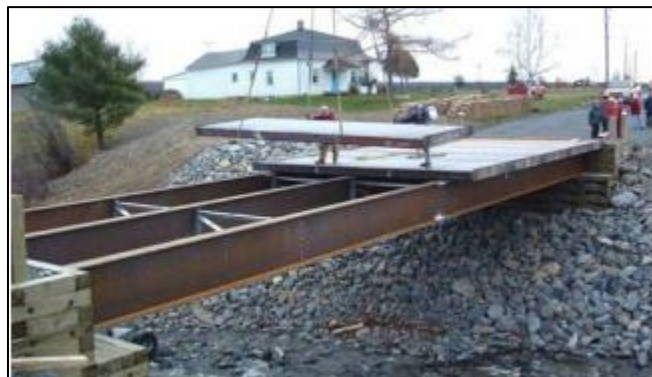
Figure 2- 14 Deck panel installation (Thomas et al. 2009)
