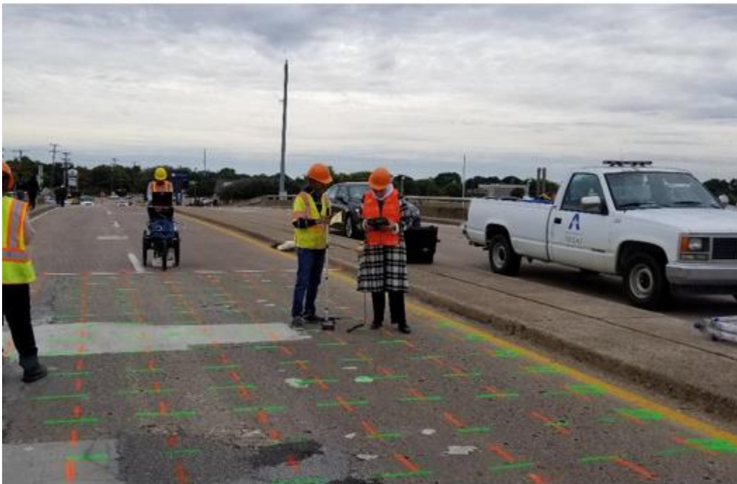
Figure 5- 4 Scanning with Cart-Mounted GPR and IE.
