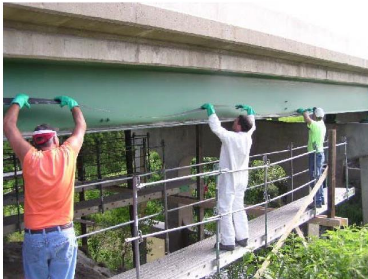
Figure 2- 16 Application of CFRP strips on girder (Iowa DOT)
