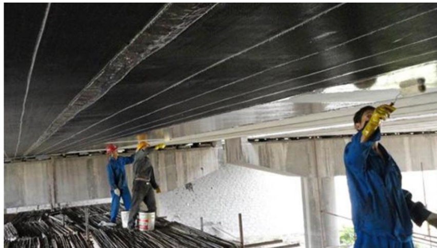
Figure 2- 10 Application of CFRP sheet (Horse Construction)
