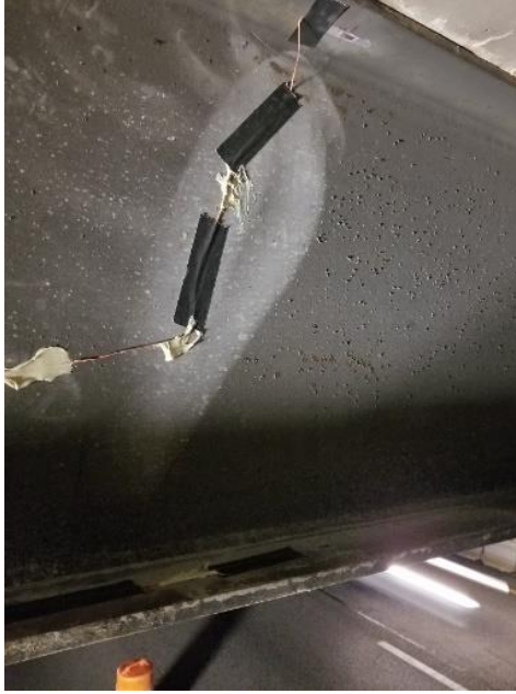
Figure 4- 1 Strain gage on the steel girder
