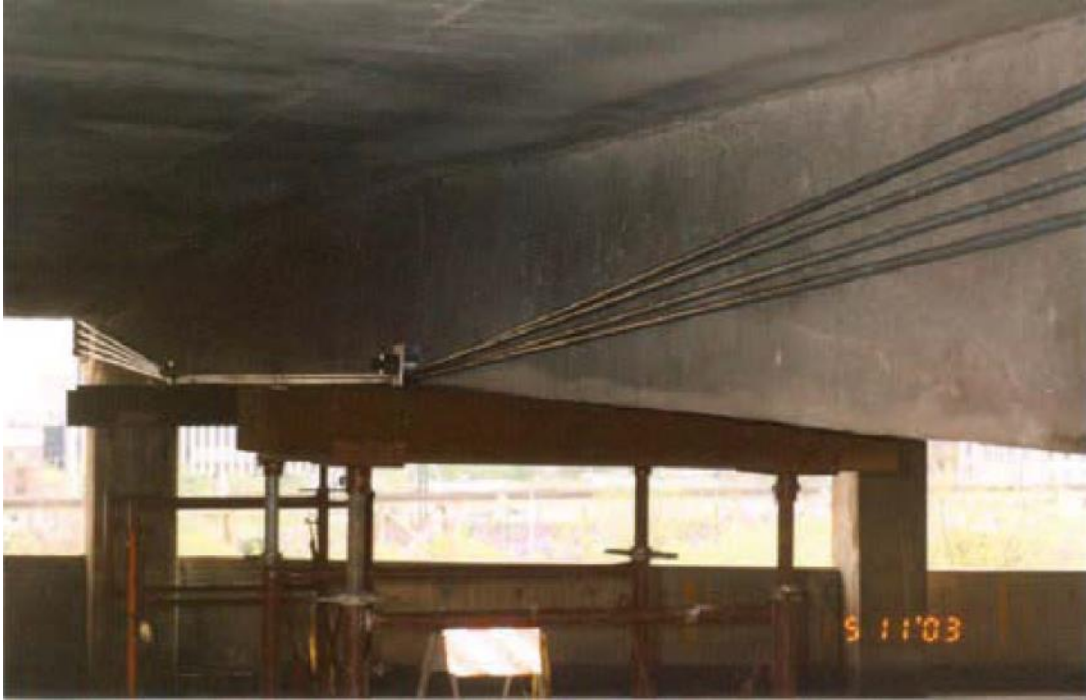
Figure 2- 18 Deviated beam strengthening tendons (Krauser, 2006)
