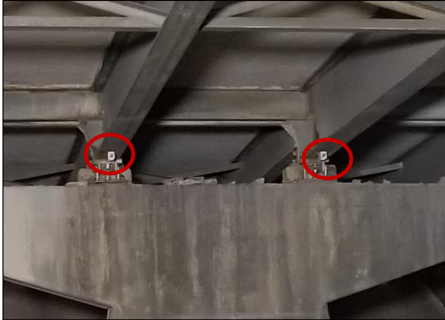
Figure 4- 8 Rotational tiltmeters at Bent 2
