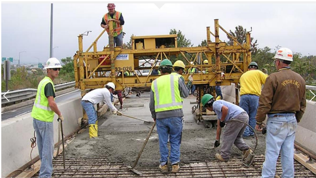
Figure 2- 9 Bridge deck rehabilitation on I 695 and Route 702 (Wagman, 2005)
