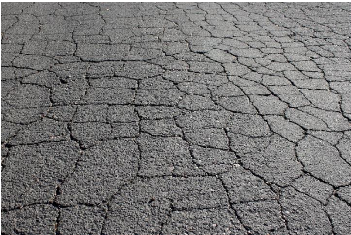
Figure 2.10. Fatigue cracking
