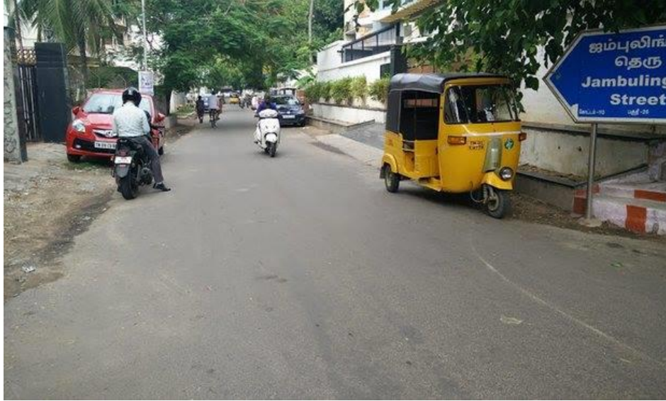
Figure 2.18. Jambulingam Street, one of India's first plastic roads (Mizikar et al, 2019)
