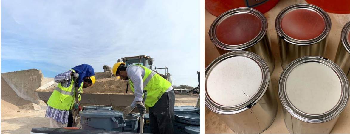
Figure 3.1. Aggregate & Bitumen collection from Austin Paving Co., Goodnight Lane, Dallas
