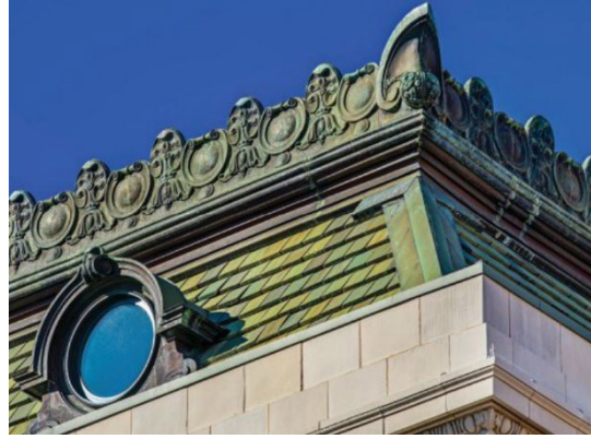
Figure 3.6 Restored green clay tile mansard roof (Lucy)
