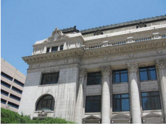
Figure 3.5 Pre-restoration appearance of the building exterior (Lucy)
