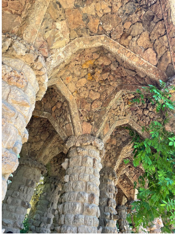
Figure 2.7: Columns in Park Güell (Fatimah, 2022)
