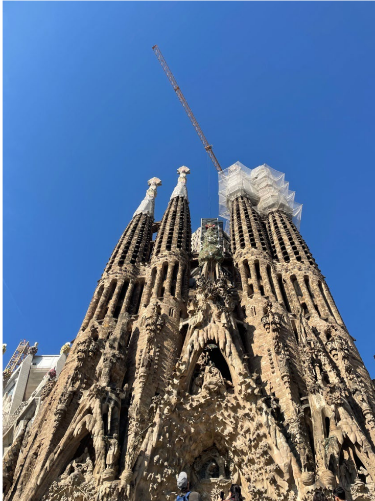
Figure 3.2: Sagrada Família Under Construction (Fatimah, 2022)
