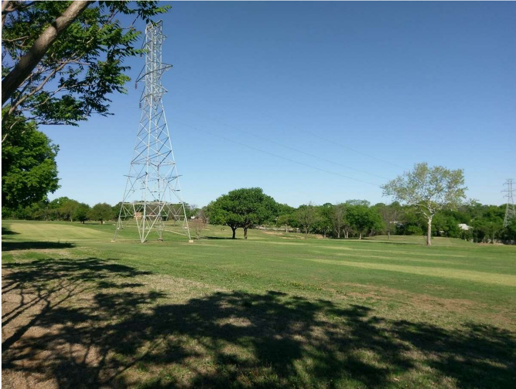
Figure 4.9 Photo by Author, Tower in 12 fairway.
