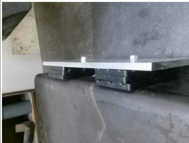
Fig. V.1 – (3)1/4" Full Bearing Shims Free Fit Holes
