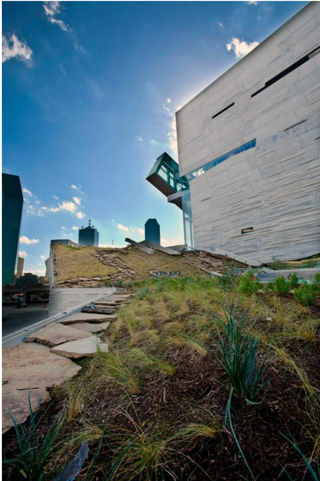
Figure 12: A portion of the plinth roof has a 1-ft vertical: 1.5-ft horizontal grade, which is a focal point for the project. Source: Talley Associates (2017)
