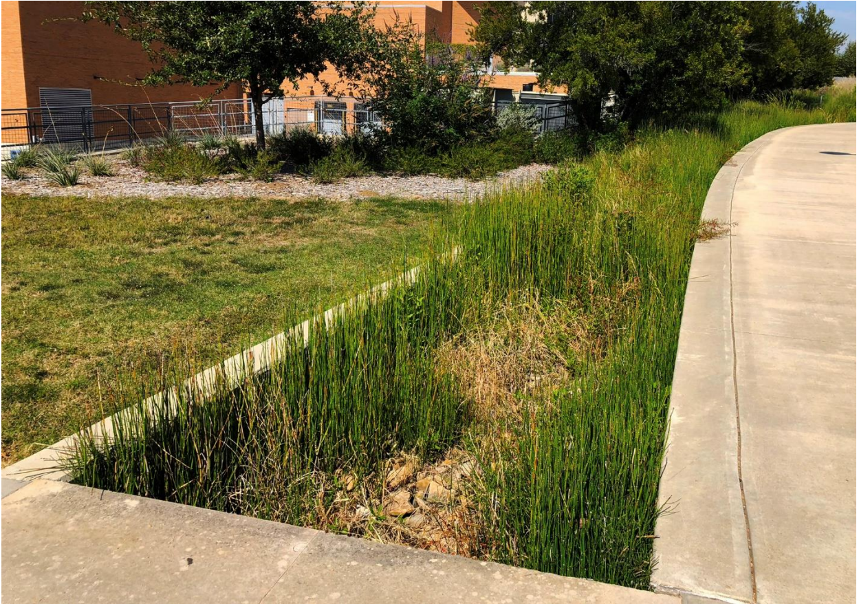
Figure 5: Three keys to the success of the stormwater design included a soil medium with high infiltration and growing characteristics, a plant palette that could withstand both dry and flooded conditions, and a ground cover material that was resistant to erosion. The horsetail reeds ( Equisetum hyemale ) in the bioswale along the western edge of the Green were used for their excellent filtering and cleansing properties. Source: Author (2017)
