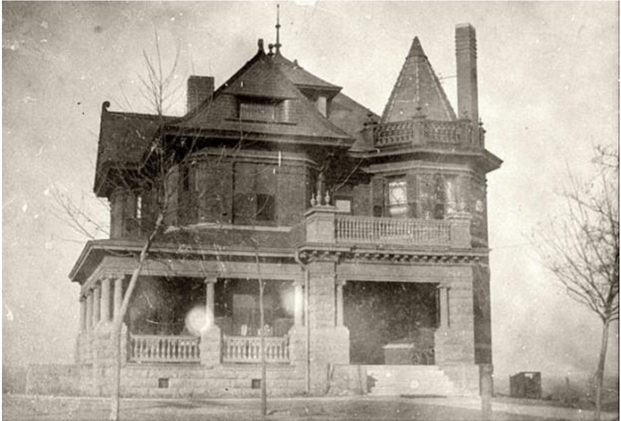
1120 Penn Street, Fort Worth. Commonly known as the Pollock-Capps House. William Capps purchased the house in 1910, and the structure would remain in the family's possession until 1971. The building is currently home to Dent Law Firm. This photograph, probably taken in 1900, is found in The Tarrant County Historical Journal 3, no. 1 (spring 1997), 16.
