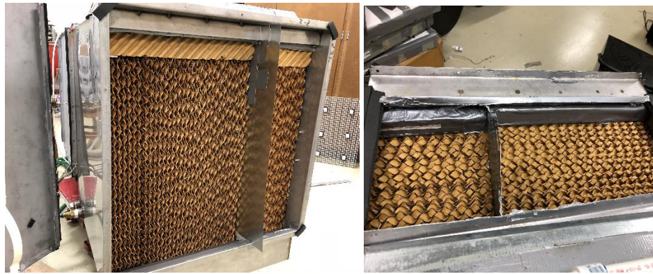
Figure 3-2 shows Side and top view of the DEC pad fitted inside the middle duct.
