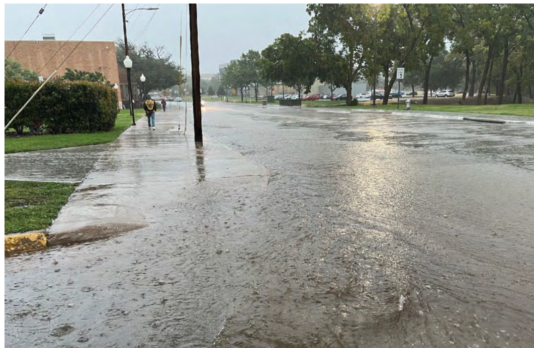
Greek Row flooding corrections; stormwater contained largely in right of way after improvements (Source: UTA)
