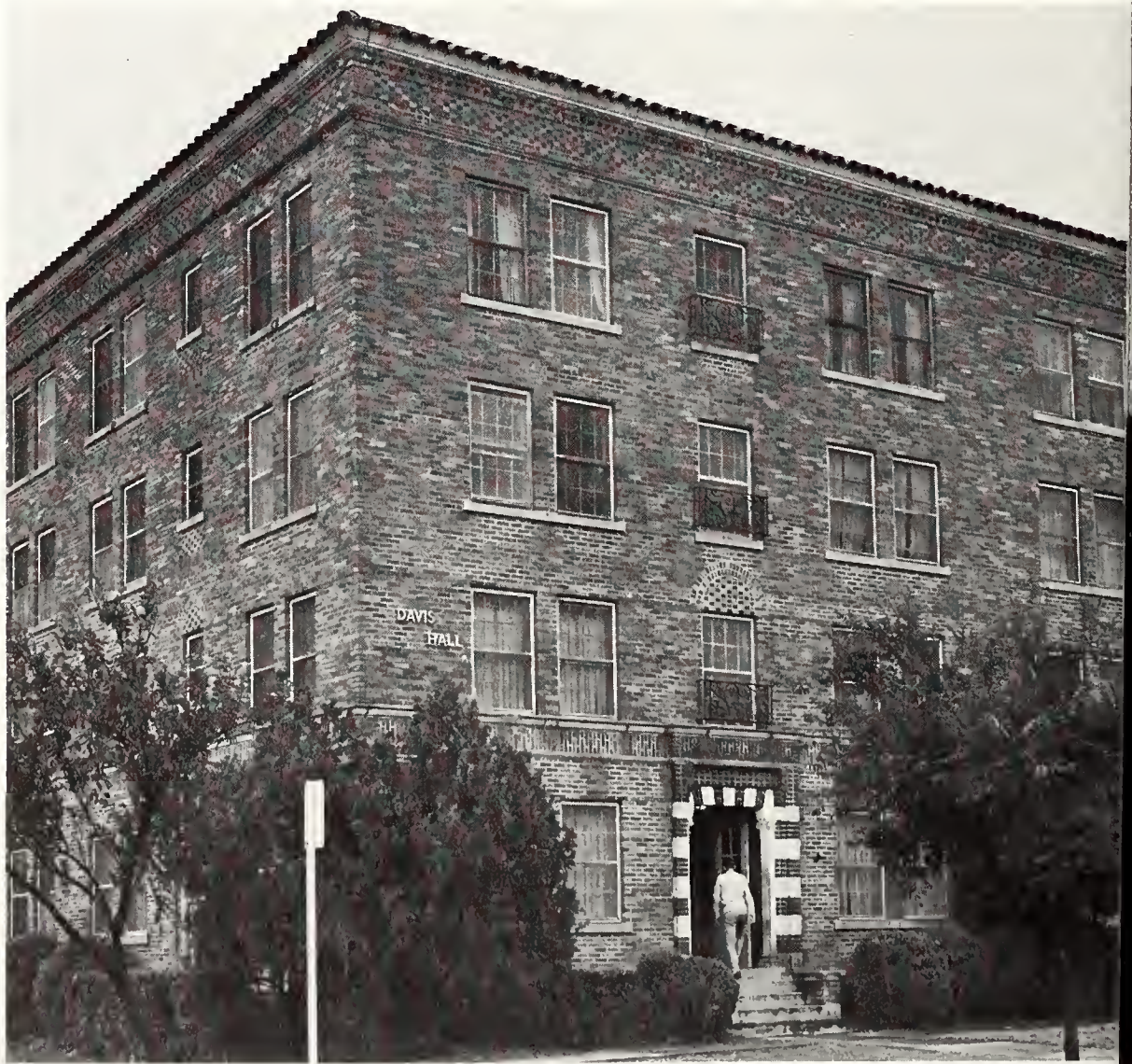
Davis Hall for boys is the oldest dormitory on campus.
