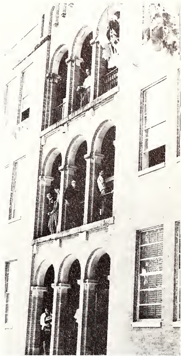
Balconies of the Administration Building provide a vantage point for the people-watchers on campus.
