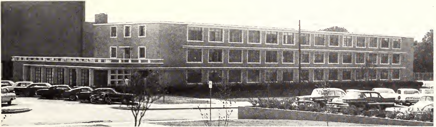
Pachl Hall, located next to Texas Hall and Trinity Dorm, sports a sun deck on the second floor for the use of its 144 residents.
