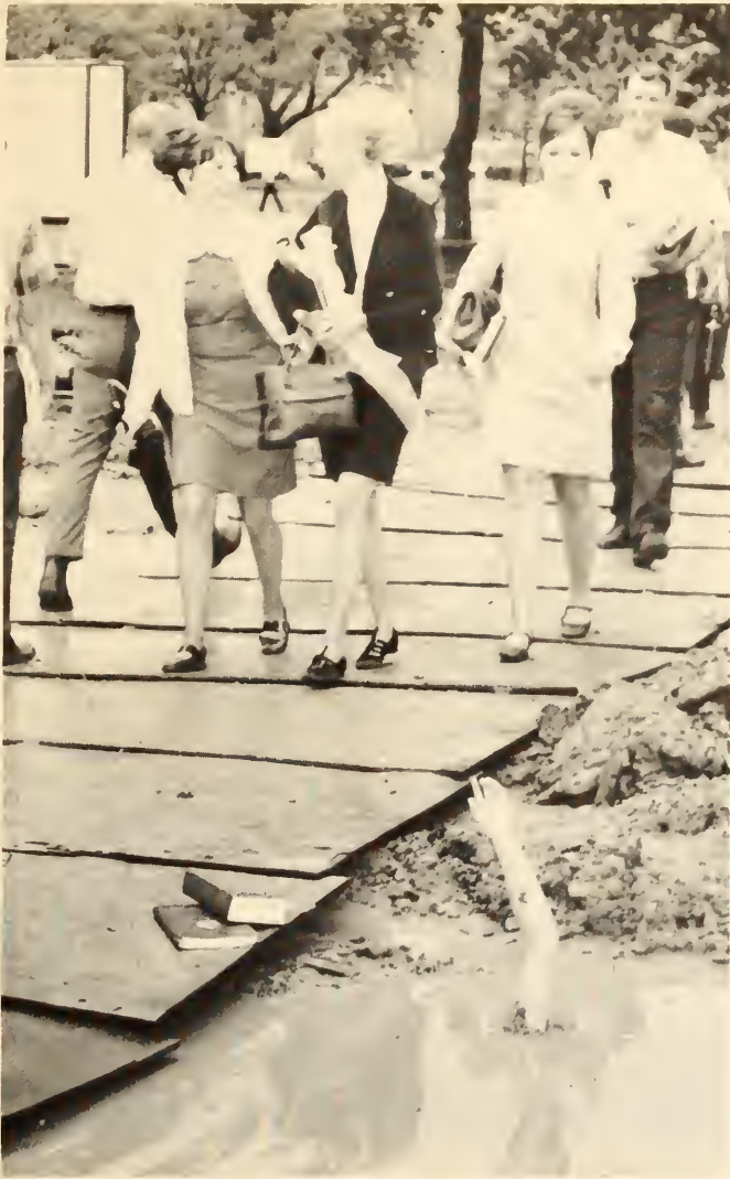
Construction problems caused by bad weather turned the campus into a stream laced bog, with mud-covered boards serving as sidewalks.
