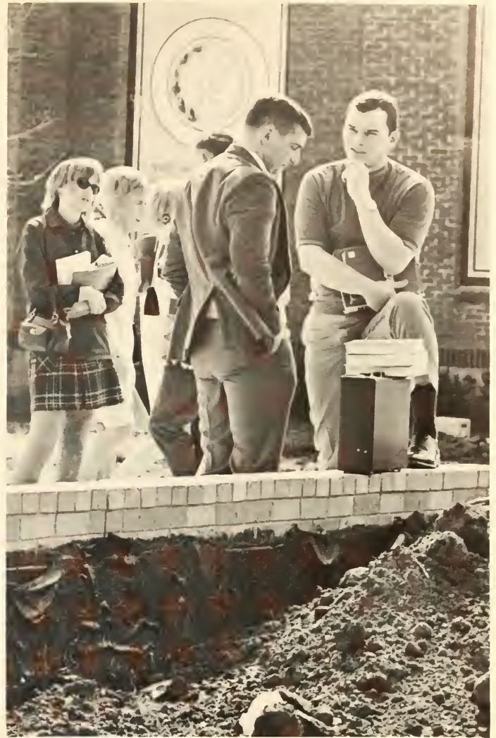
Brick planters being constructed on the mall provide place for conversation.
