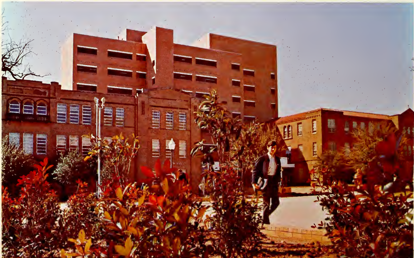
Carlisle Hall rises above the Administration Building and Preston Hall, both long-time landmarks.
