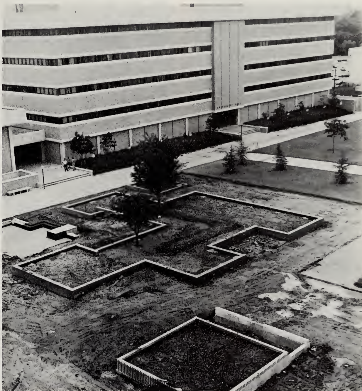
UPPER LEFT: One way traffic prevails on wooden 2 by 4's laid to allow clean passage over muddy stretches. FAR LOWER LEFT: Workman works on new fuel storage tank. LOWER LEFT: Pipe stacks up as building gets underway. TOP: Workers lay endless rows of decorative brick on the new mall. ABOVE: Skeleton of new mall looms out of mud.
