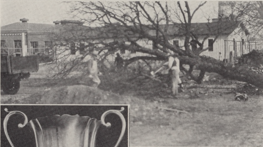
2. Making way for the new gym.
