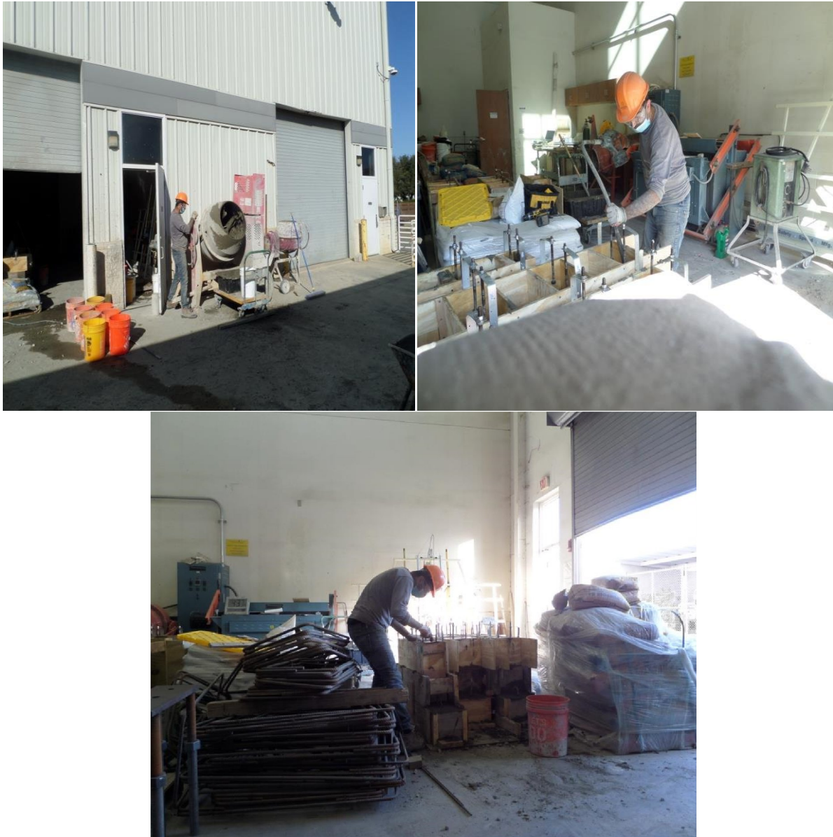
Figure 3.16 On-Site Concrete Mix
