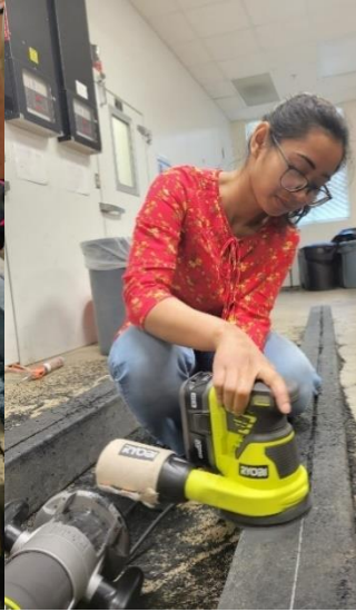
(b) Sanding for a smooth surface
