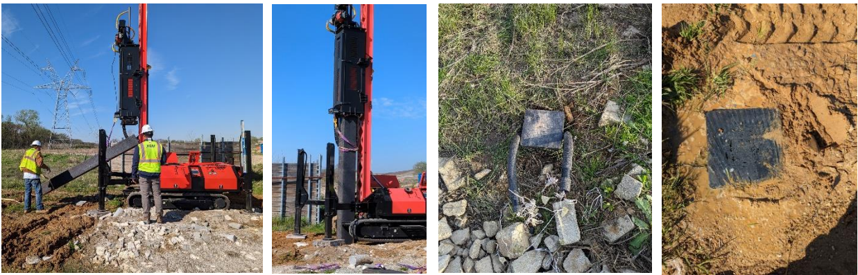
Figure 3-7 Field Installation of 25 cm × 25 cm, and 30 cm × 30 cm RPPs
