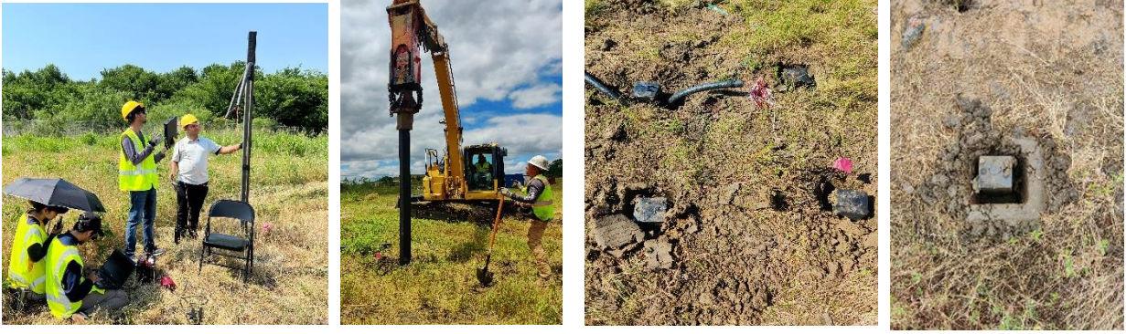
Figure 3-6 Field Installation of 10 cm × 10 cm, and 15 cm × 15 cm RPPs
