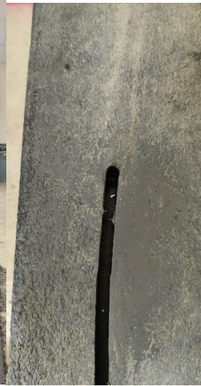
(c) Grooved and sanded surface
