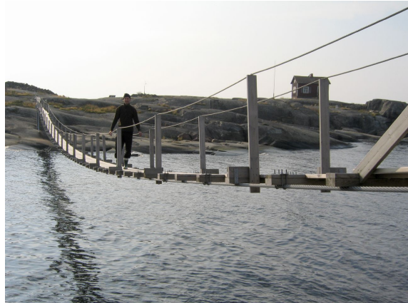
(b) Hanging bridge
