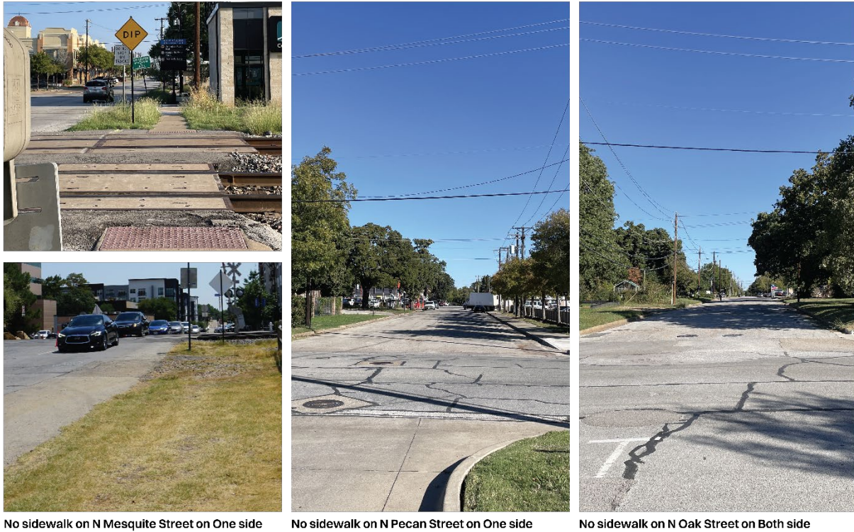
Figure 25 Existing No Sidewalk Conditions Around the Design Site
