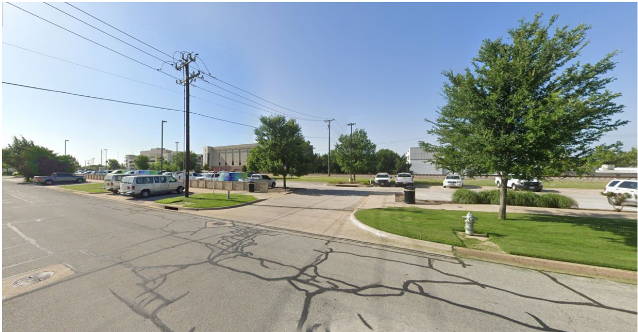
Figure 41 Existing Condition of the Intersection on Pecan Street and Front Street (Source: Google Maps)
